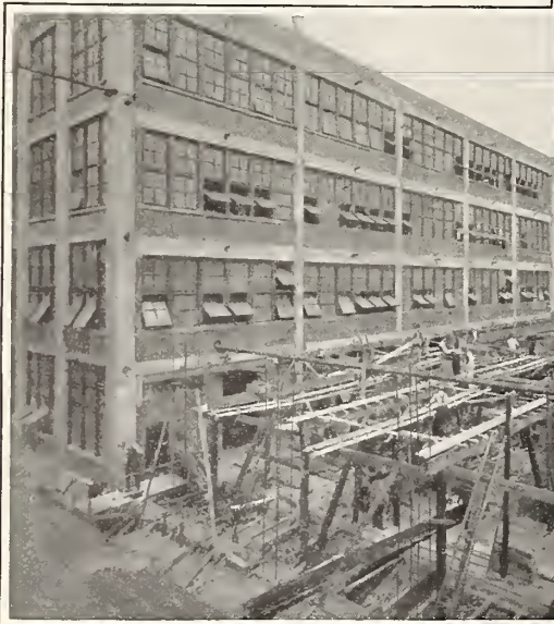
EXTENSION TO NEW VICTOR CABINET FACTORY.
