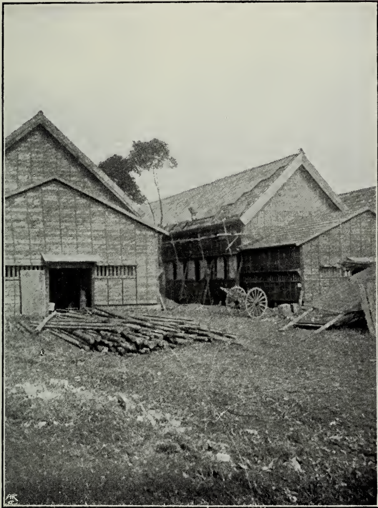
VIEW OF HUT IN COURSE OF CONSTRUCTION (JULY 1904).
