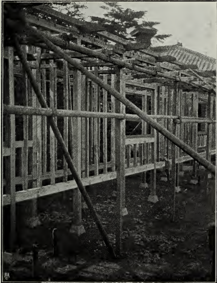
VIEW OF FRAMEWORK OF CORRIDOR IN COURSE OF CONSTRUCTION (JULY 1904).
