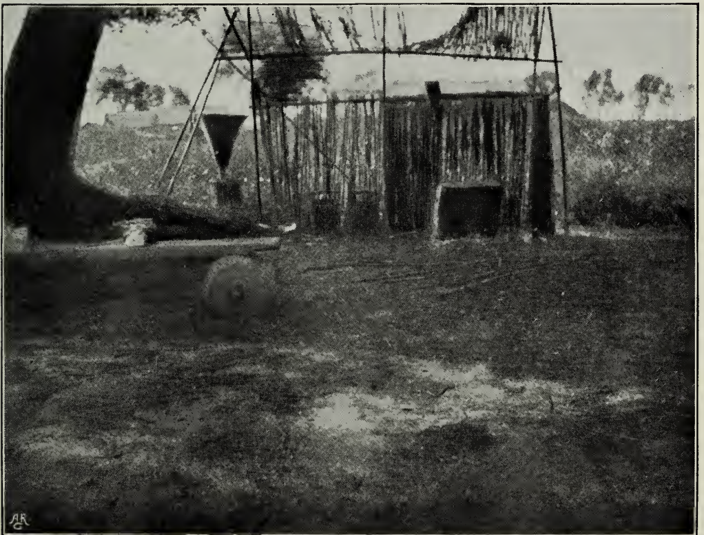
Station for boiling water at Tang-hsiang-kung-tai, during summer of 1905, showing field kitchen and rice cauldron for boiling the water, with the Ishiji filter for clarifying the water beyond.
