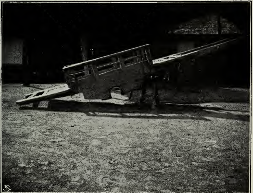
Body of cart of photograph 9, showing the bearings of the axle. These photographs are intended for the purpose of illustrating the absence of springs or other contrivance for the prevention of jolting.
