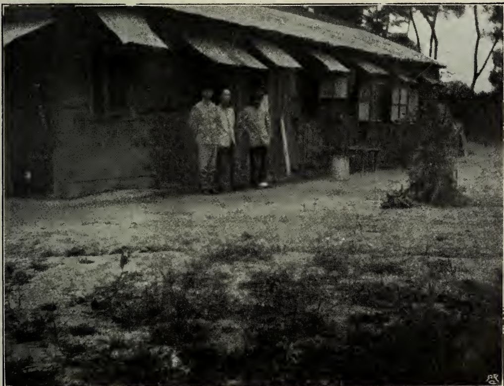
Laboratory building at the head of the line of communication of 2nd Army, Ching-yun-p'u, summer of 1905. It is erected in the garden of the house used by the Principal Medical Officer of the line of communication, and was equipped for chemical and bacteriological work,
