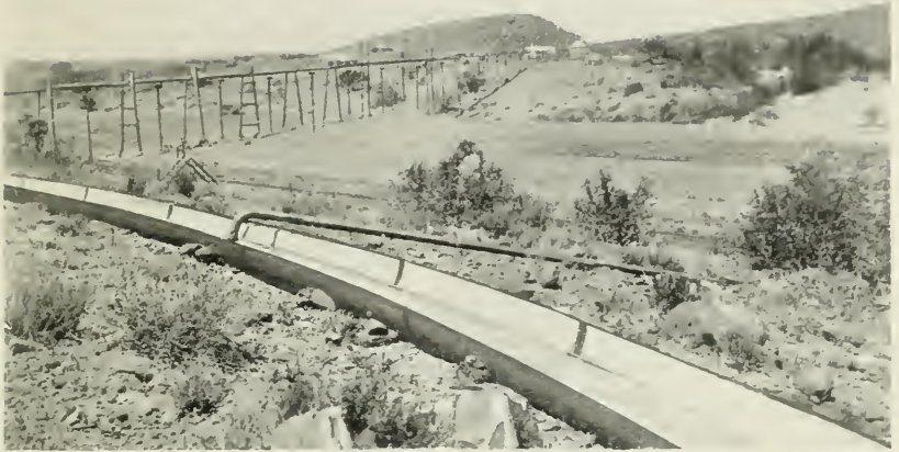
IRRIGATION : MAIN WATER FURROW AND LOCAL SYPHON
