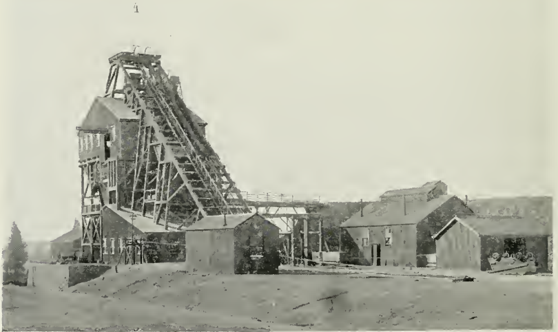
HEAD-GEAR AND SORTING HOUSE AT THE ROBINSON MINE, JOHANNESBURG
