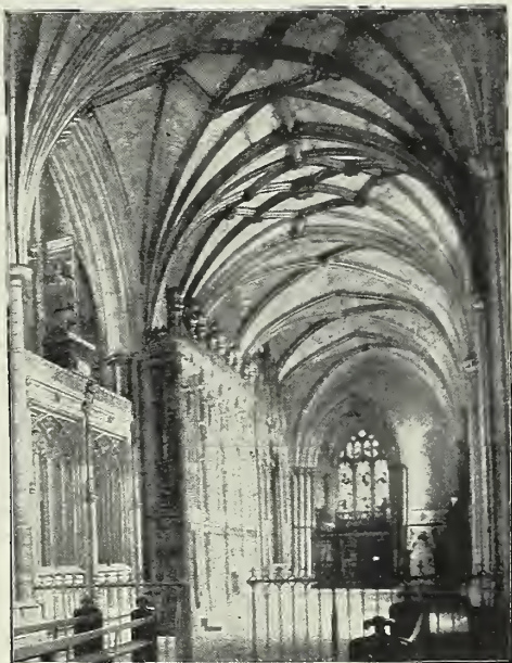
FIG. 76.—SOUTH AISLE OF WINCHESTER CATHEDRAL, ENGLAND.
