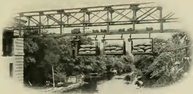
A DETAIL OF THE TELPHERAGE SYSTEM.
