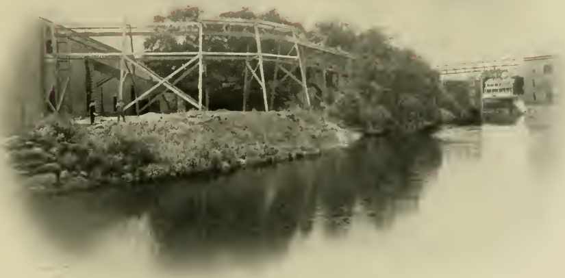
THE TELFERAGE SYSTEM — FOR THE CONVEYANCE OF CRUDE COCOA FROM THE STOREHOUSES TO THE ROASTING ROOMS.
