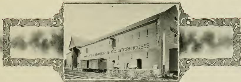
WALTER BAKER & CO.'S STOREHOUSES, MILTON.
