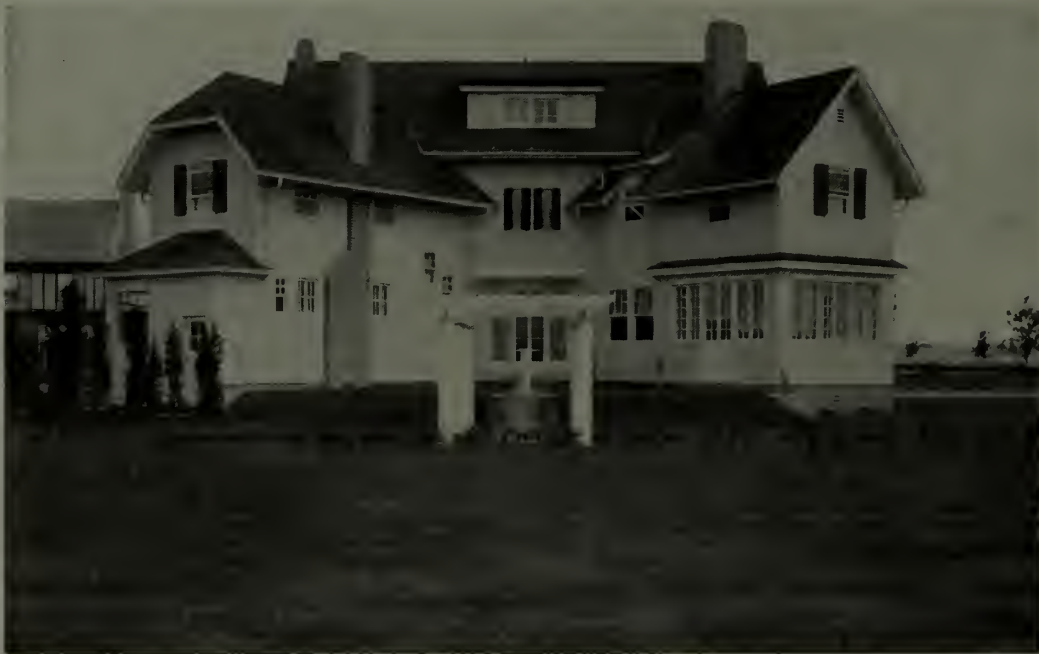
Rear view of the house showing the pergola and sundial. Note the differences in detail in the two wings. Growth of the planting will add greatly to the general effect
