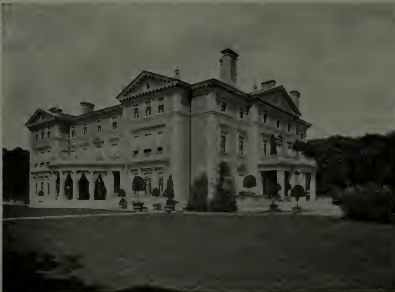
The house itself is an imposing three-story structure of brick with stone trim in the style of the Italian Renaissance
