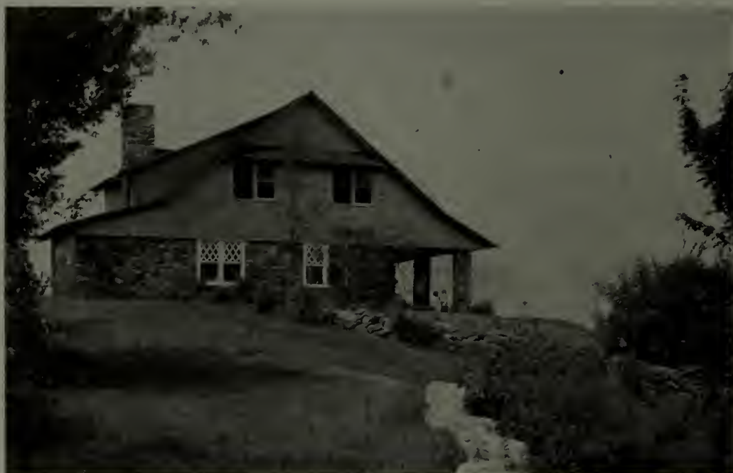
The house is low and broad, the first story of native field stone serving to tie it to the soil and make it seem a component part of its environment. East end of the house from the highway
