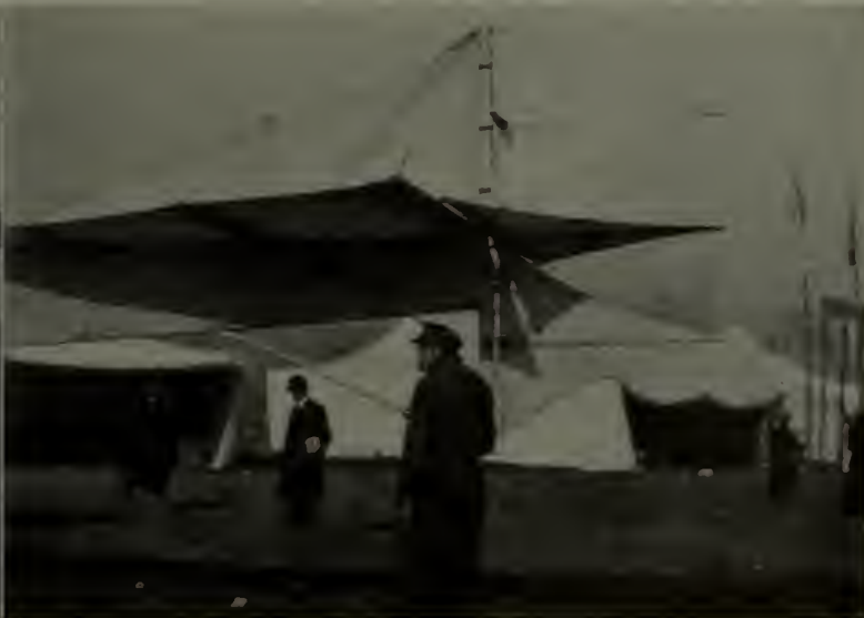
The tail and steering gear of the Antoinette are made up of movable triangular sails, and the whole somewhat resembles the feathered tip of an arrow
