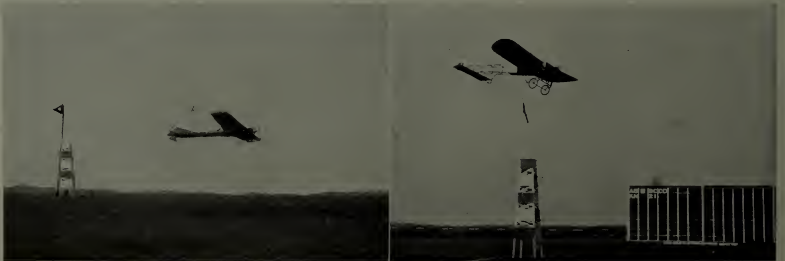
Hubert Latham flying in his 16-cylinder, 100-horsepower Antoinette monoplane at Belmont Park last October. The Bleriot type of monoplane, flown by the late John B. Moisant. This form approaches as near to the scientist's ideal as any
