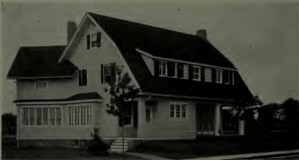
View of front and south side of the house, showing how the entrance hall divides the entrance porch from the porch proper, giving a measure of seclusion to the latter
