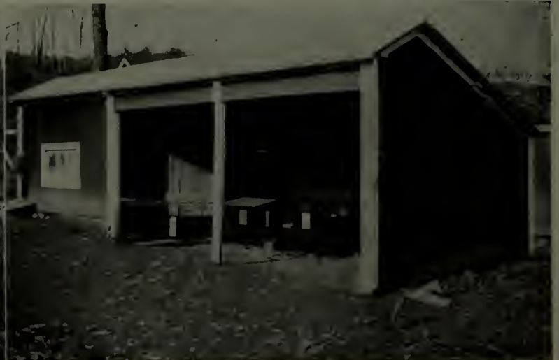
Brooder house. The brooder under the shed is for small chicks just from the incubator. The enclosed part of shed has bottom heat and is for larger chicks
