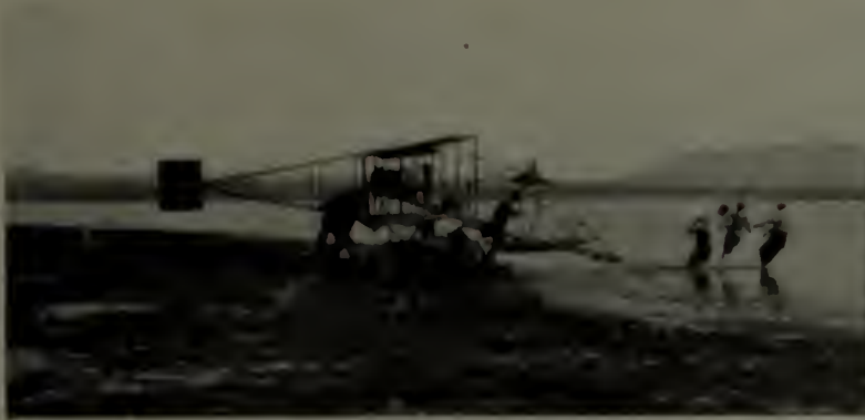
Hauling the machine down from the barge
