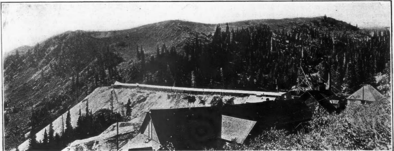
Hoisting plant at Judge shaft
