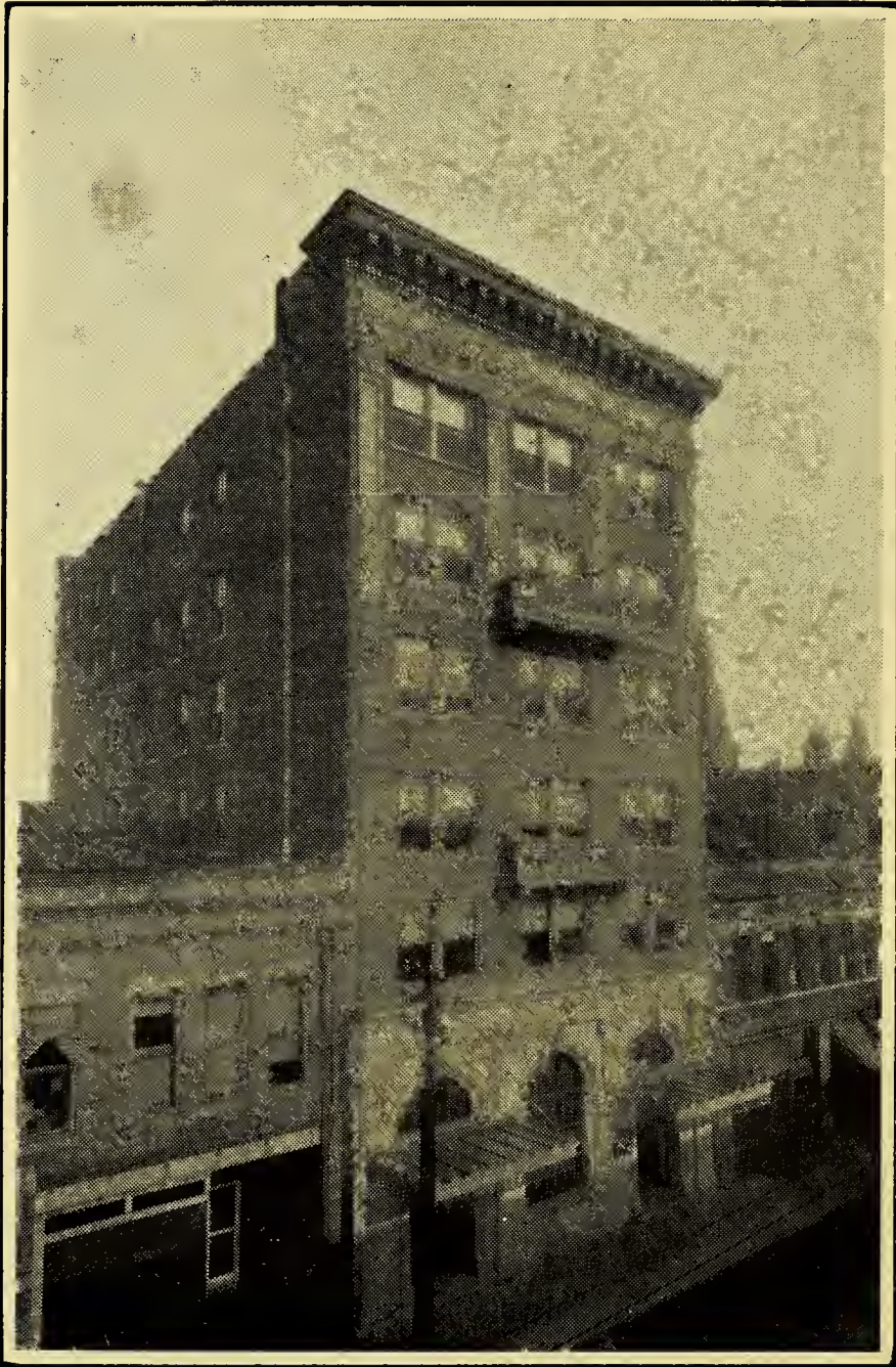
HOME OFFICE BUILDING N. C. MUTUAL LIFE INS. CO.
