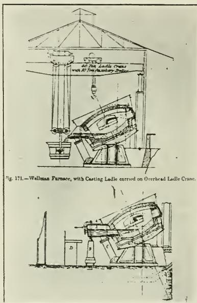
Fig. 171.—Wellman Furnace, with Casting Ladle carried on Overhead Ladle Crane.
