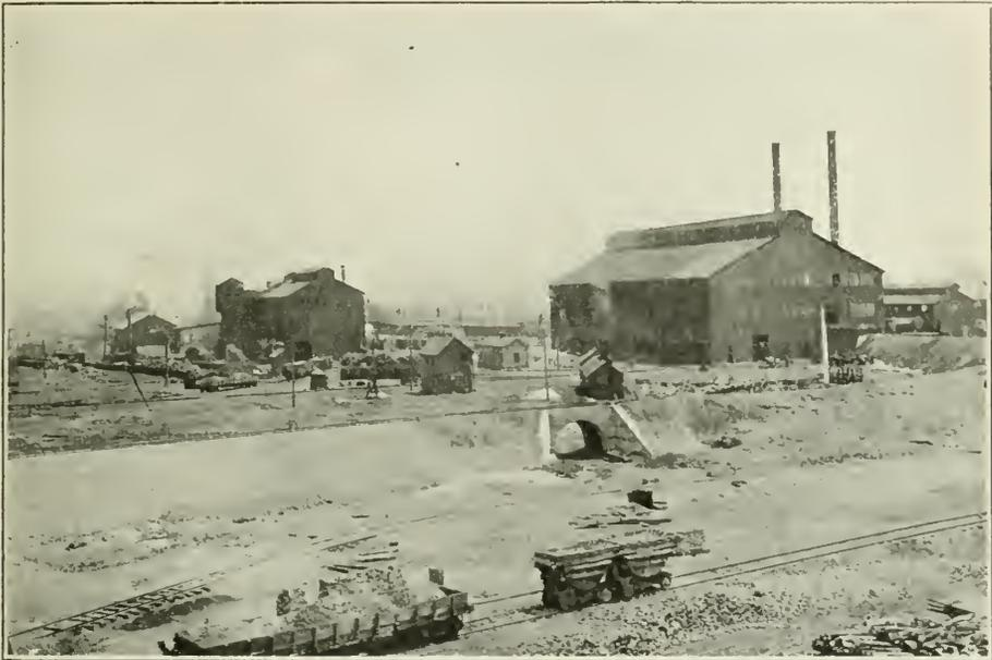
Algoma Steel Company. Basic open hearth building on the right; bessemer plant and rail mill on the left.
