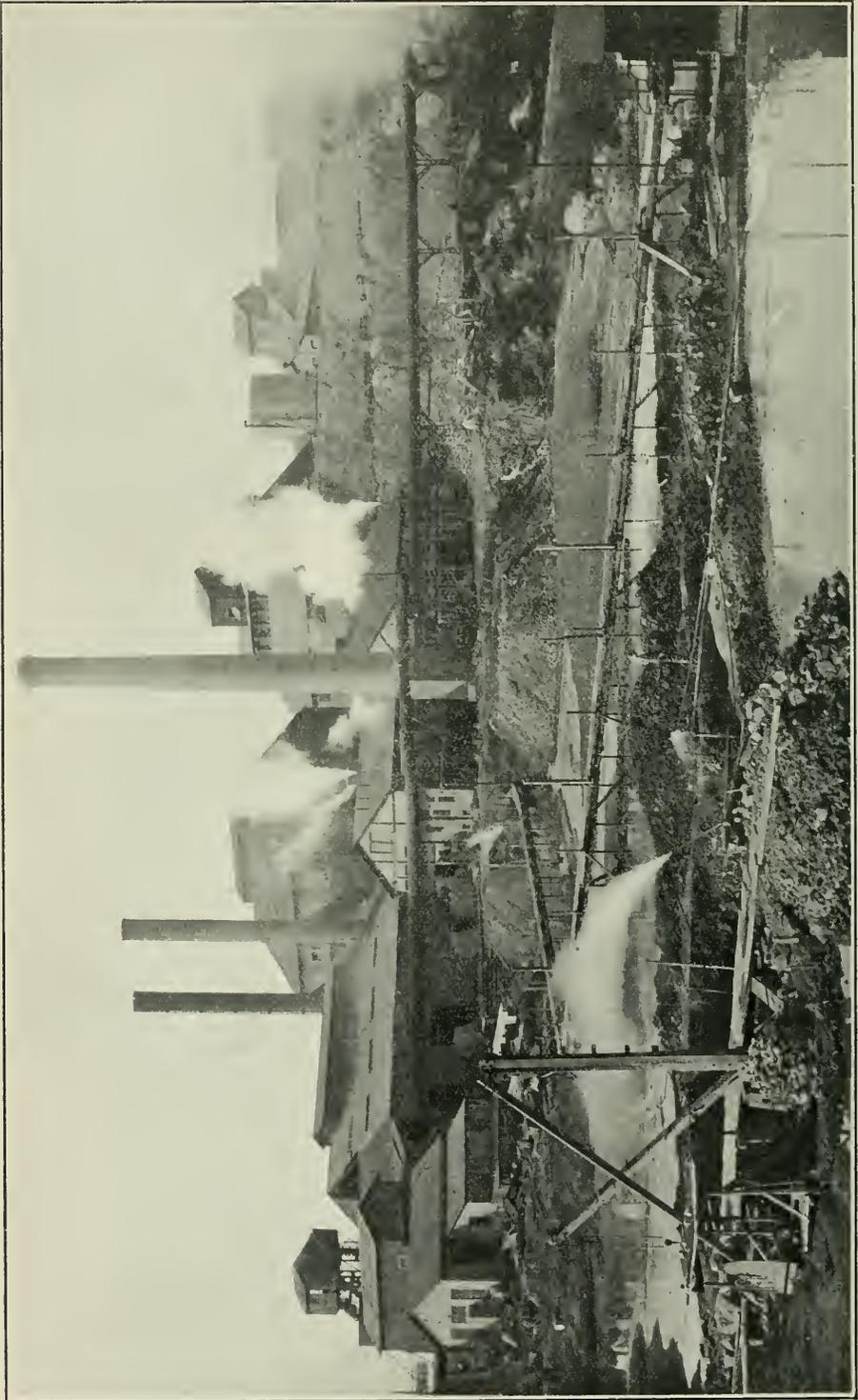
View of concentrating and nodulizing plant at Lebanon, Pa.; magnetic separators in upper portion and nodulizers in lower portion of mill. *U.S.G.C.*
