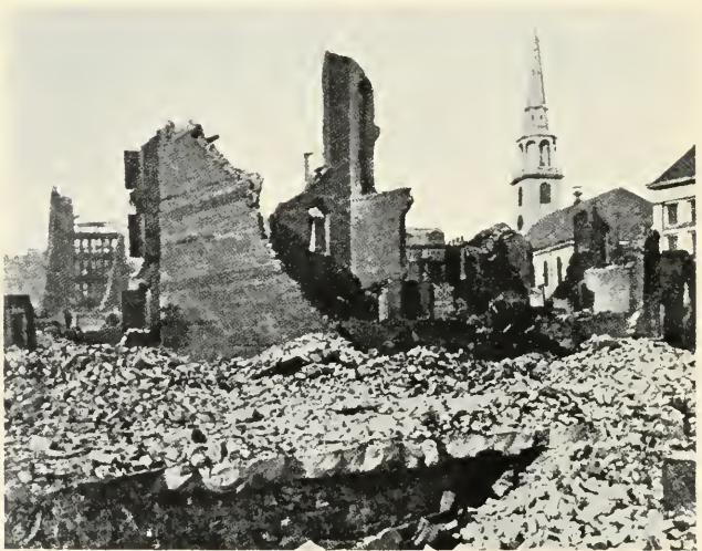
ANOTHER VIEW OF THE FIRE RUINS.
