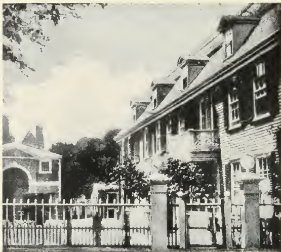
LEONARD VASSALL HOUSE, SUMMER STREET, THE SITE OF HOVEY'S STORE.
