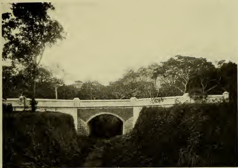
SIDE VIEW OF "EL ROTULO" BRIDGE
