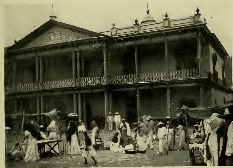
BARRACKS AT COJUTEPEQUE, DEPARTMENT OF CUSCATLÁN.
