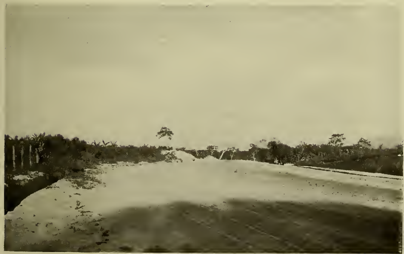
THE FAMOUS AVENIDA UNDER CONSTRUCTION.
