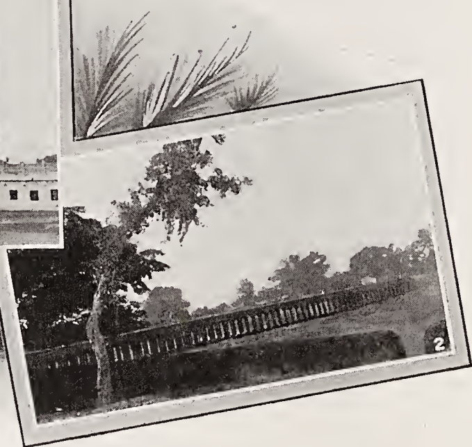
2. BRIDGE AT SERINGAPATAM.
