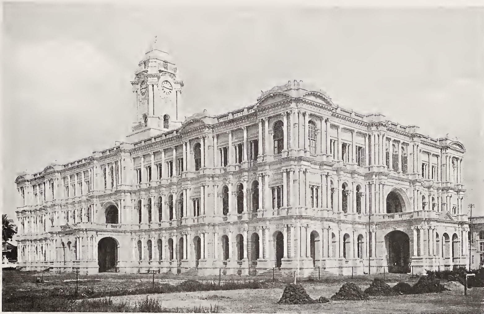
RIPON BUILDINGS, MADRAS, BUILT BY P. LOGANATHA MUDALIAR.
