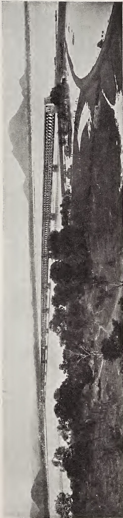
KISTNA BRIDGE, M. & S.M. RAILWAY.
