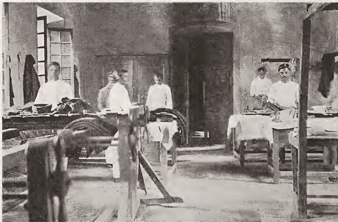
T. G. BAILEY & CO. DYE-HOUSE AND FINISHING-ROOM.
