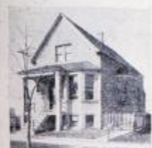
A No. 2128 IDEAL Boiler and 270 ft. of 38-inch AMERICAN Radiators, costing the owner $135, were used to Hot-Water heat this cottage.
