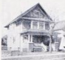
A No. A-221 IDEAL Boiler and 466 ft. of 38-inch AMERICAN Radiators, costing the owner $215, were used to Hot-Water heat this cottage.
