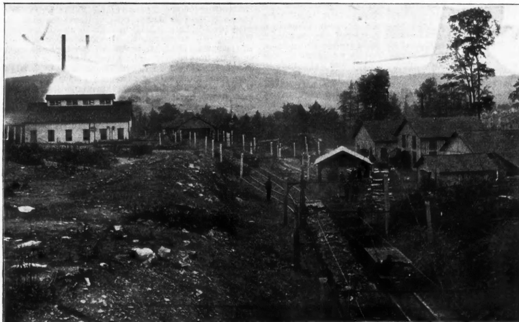
VIEW ABOVE ENTRANCE TO EUREKA MINE NO. 30.
