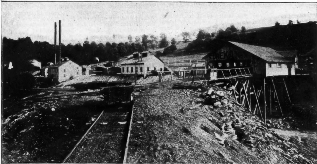
POWER STATION AND TIPPLE, UREKA MINE NO. 31.
