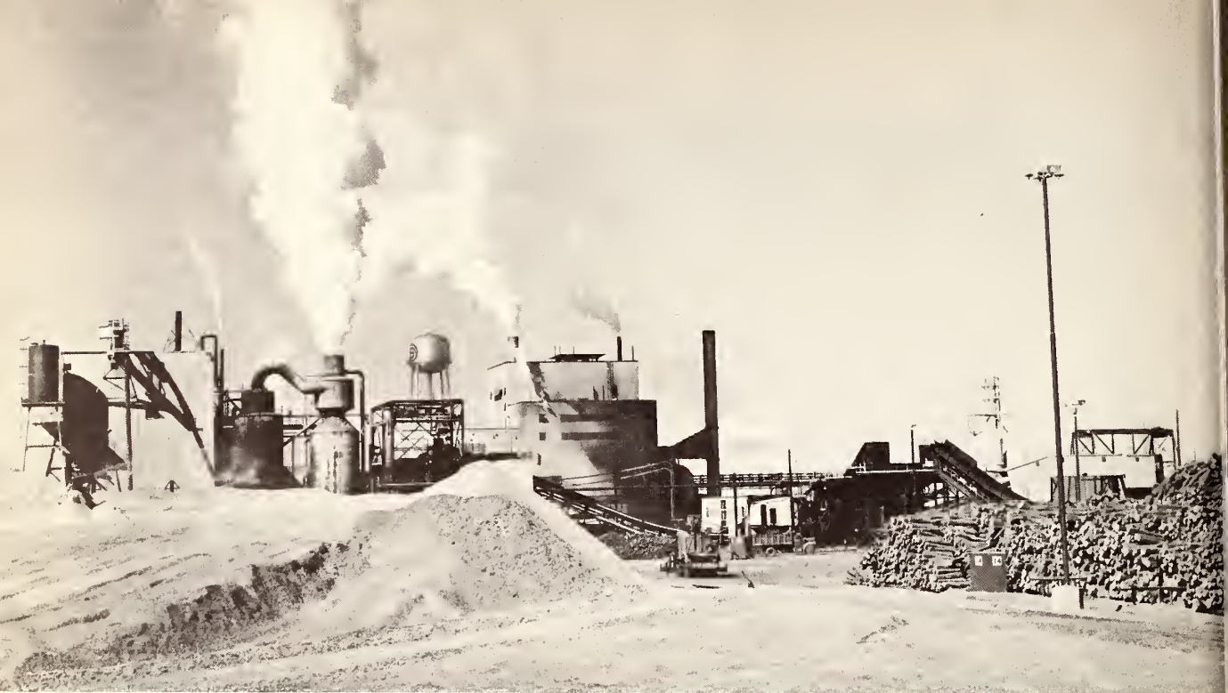
Figure 23. --The Southwest Forest Industries, Inc., pulpmill near Snowflake, Arizona, uses underground water entirely in the manufacturing process. This mill produces about 165,000 tons of Kraft linerboard and newsprint per year using round pulpwood and chipped sawmill residues (foreground).
