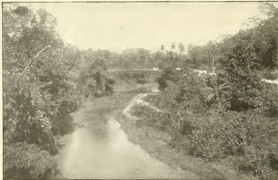
BRIDGE ON RIO COBRE RIVER.
