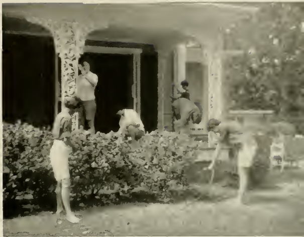
Tri Deltas make repairs.
