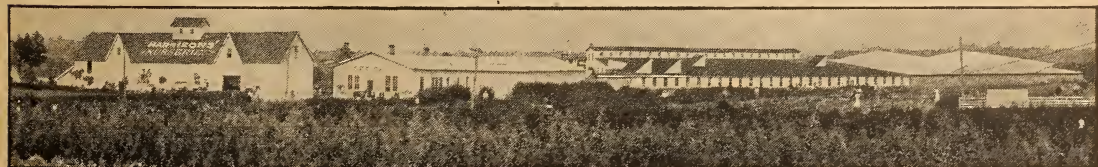
General View of Harrisons' Modern Packing House with Up-to-Date Facilities Which Enable Us to Properly Grade, Pack and Ship Thousands of Packages of Harrison Grown Products Daily
