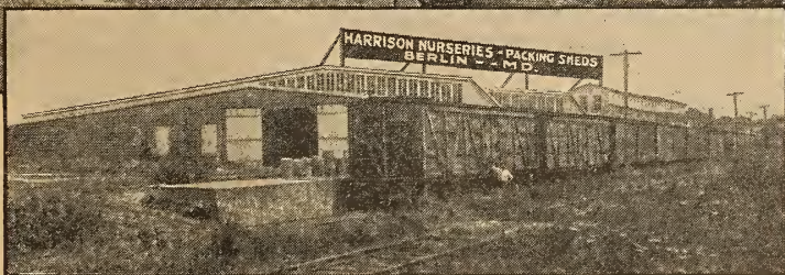
Side View of Packing Houses with Private Railway Siding Holding 35 Freight Cars
