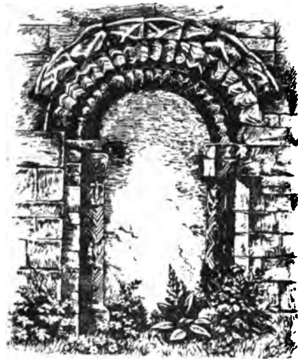
OLD SOUTH DOORWAY.
