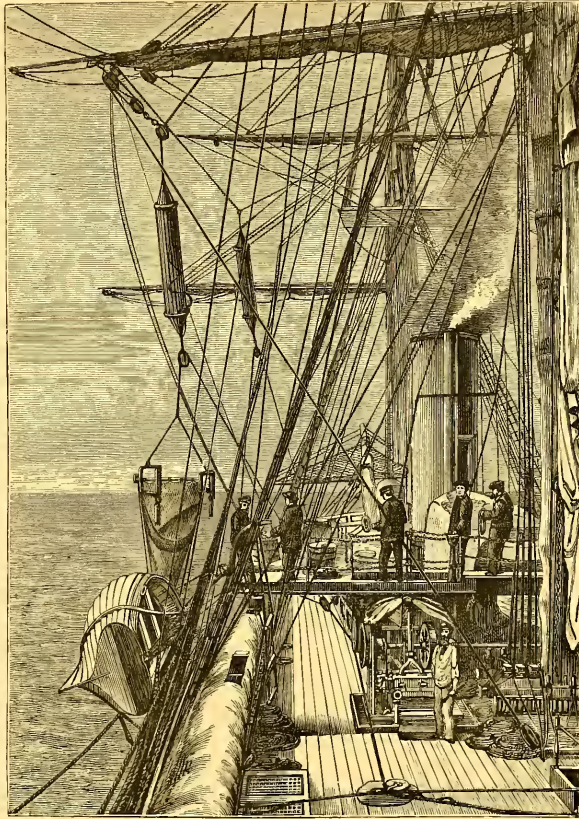
FIG. 7.—The Dredging and Sounding Arrangements on board the CHALLENGER.
