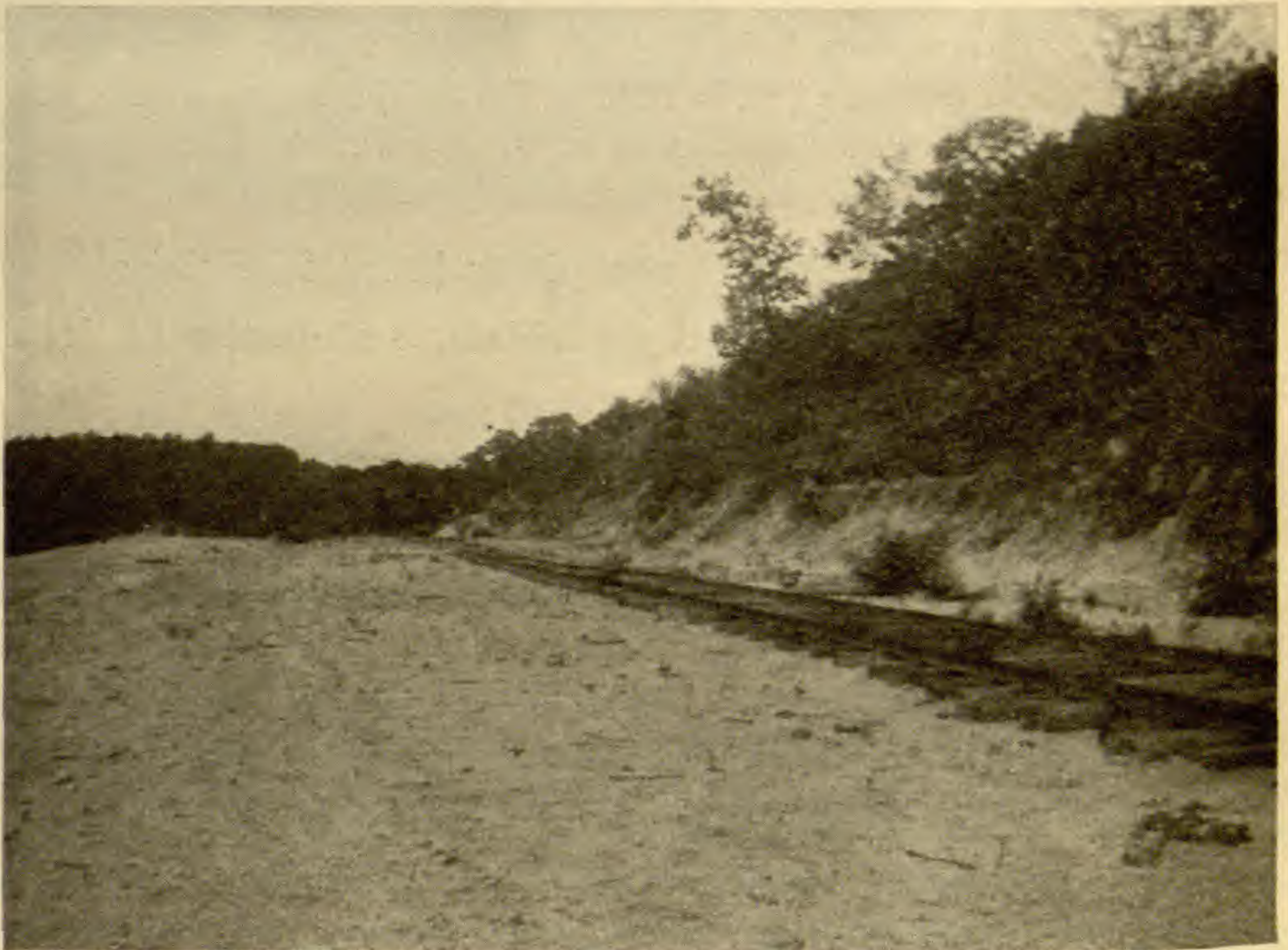
FIG. 1.—A wide level shelf for the track
