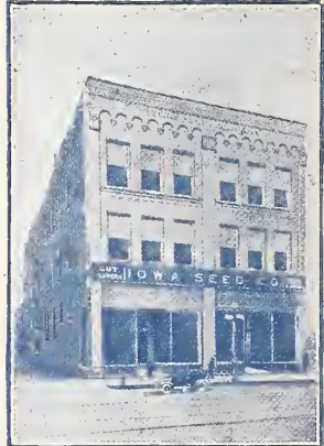
RETAIL STORE AND OFFICE 209-211 WALNUT STREET
