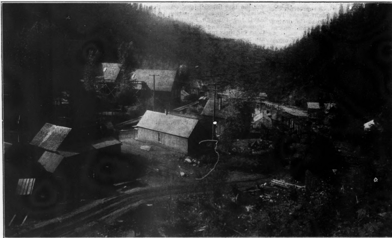
TAMARACK & CUSTER CONSOLIDATED MINING CO.'S PLANT, SUNSET, IDAHO, THREE MILES FROM WALLACE
