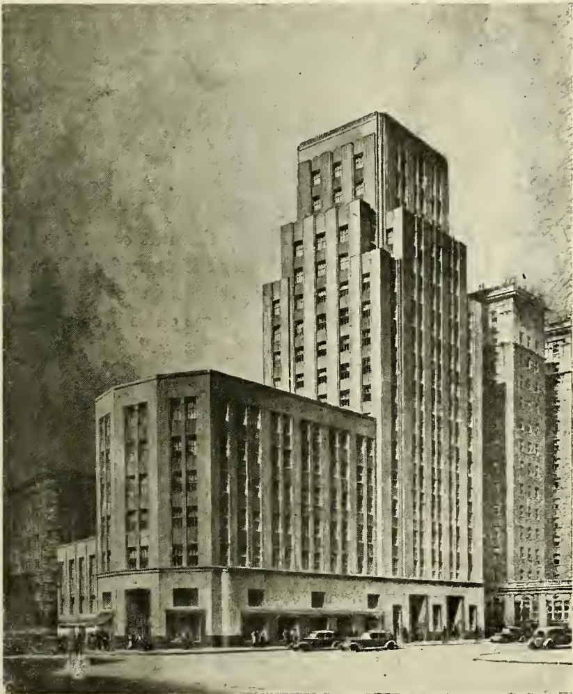
View of One Eleven Corcoran Street, Constructed at a Cost of $1,000,000, in the Heart of Durham's Business District
