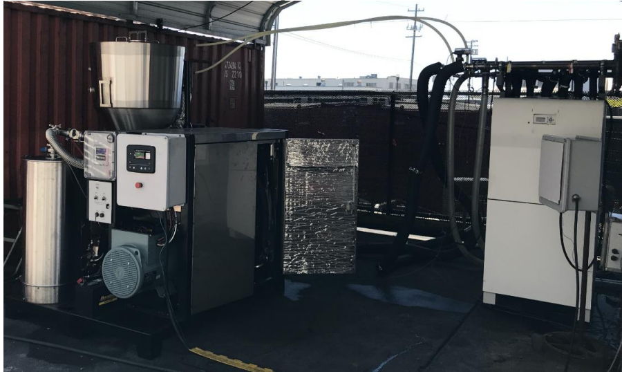
Figure 16: Final Combined Cooling, Heating, and Power Power Pallet PP1097 with Adsorption Chiller
