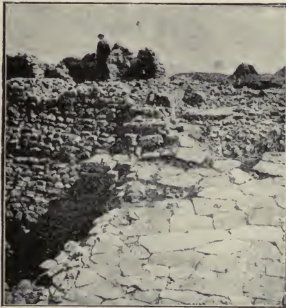
FIG. 6. PAVED RAMP AT GATE FM (II STRATUM)
