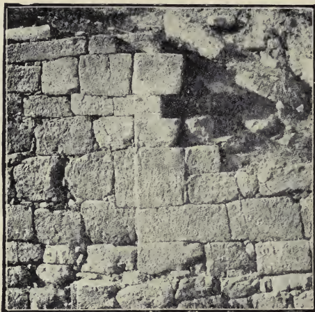
FIG. 9. RETAINING WALL OF VI M
