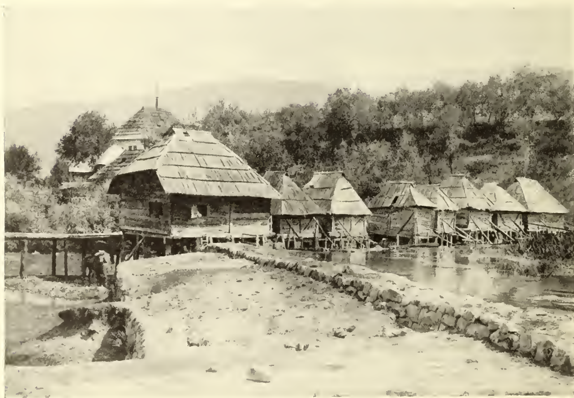
507 MILL HOUSES AT ILIDŽE
