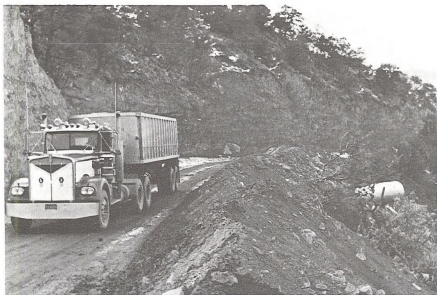
Figure S2-5. Cut-and fill construction along a road -- Loma project
