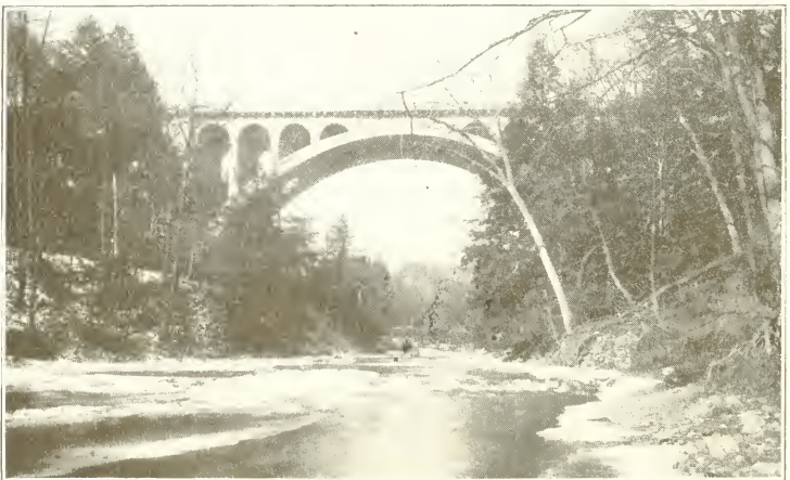
Walnut Lane Bridge across the Wissahickon
