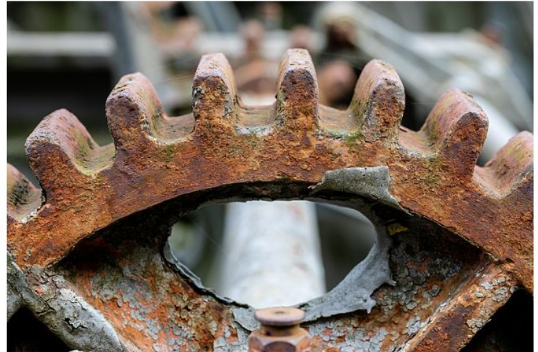
Detail of the security barrage in the Alte Fahrt of the Dortmund-Ems Canal near Greven (or Münster-Gelmer), North Rhine-Westphalia, Germany
