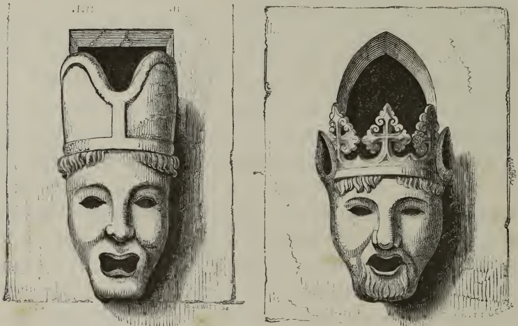
Openings in the Hall, Great Chalfield.
