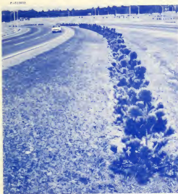
Evergreen trees planted on a curve provide a screen for headlights and safety for night driving; they serve as a beauty spot in daytime.
