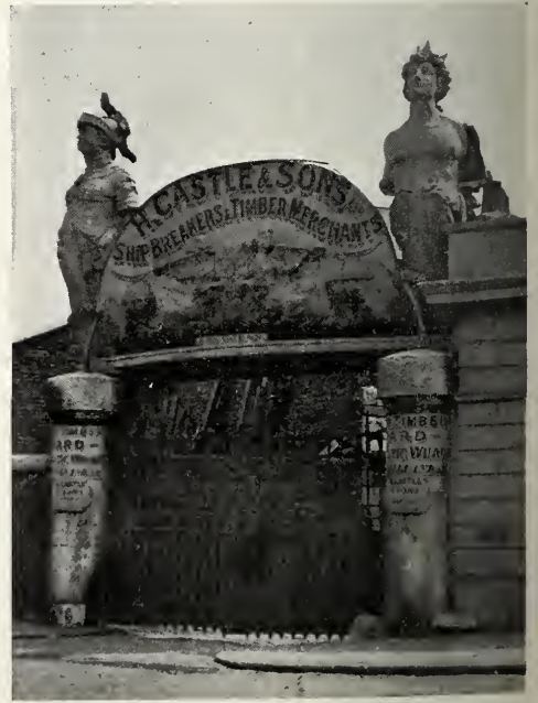
Messrs. Castle and Sons, Baltic Wharf, London, Main entrance
