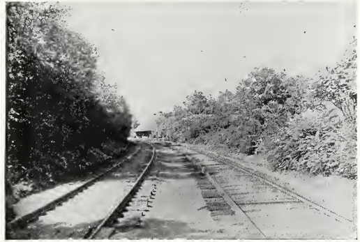
Figure V. Newton Highlands: Railway station in distance
