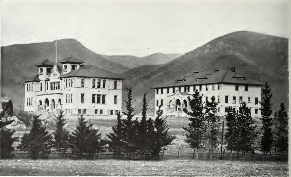
Figure XIV. The two already completed buildings of the California State Technical School, San Luis Obispo, California
