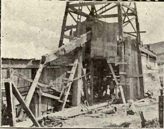
SPUDDING WELL, McDONALD OIL FIELD.
