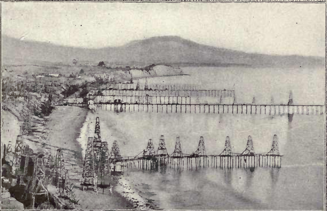
OPERATING OIL WELLS IN THE OCEAN, NEAR SANTA BARBARA, CALIFORNIA.
