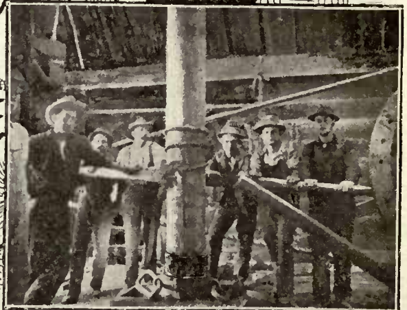
CASING WELL CALIFORNIA OIL FIELD
