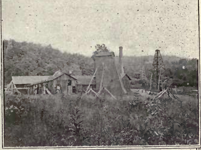
POWER HOUSE ON THE FINLETTER LEASE, HEAVY OIL DISTRICT NEAR FRANKLIN PA. IT FURNISHES POWER FOR 75 WELLS
