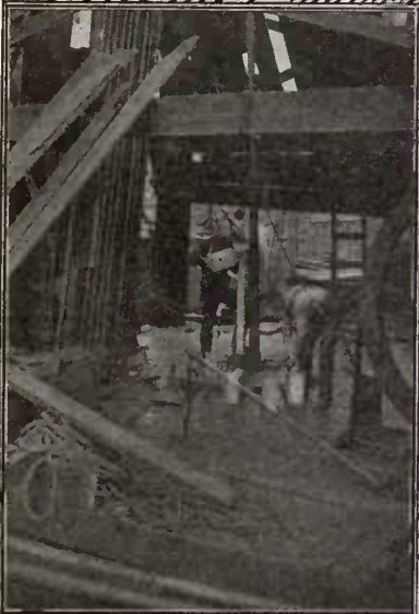
FILLING SHELL WITH NITRO-GLYCERIN MCDONALD PA OIL FIELD.
