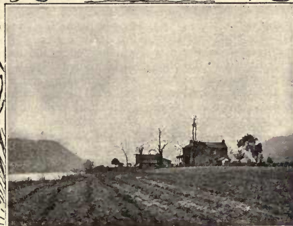
SITE OF BURNING SPRINGS KANAWHA CO. WEST VA.
