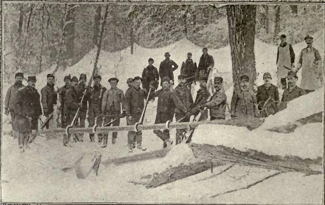
LAYING PIPE LINE NEAR OIL CITY, PENNA.
