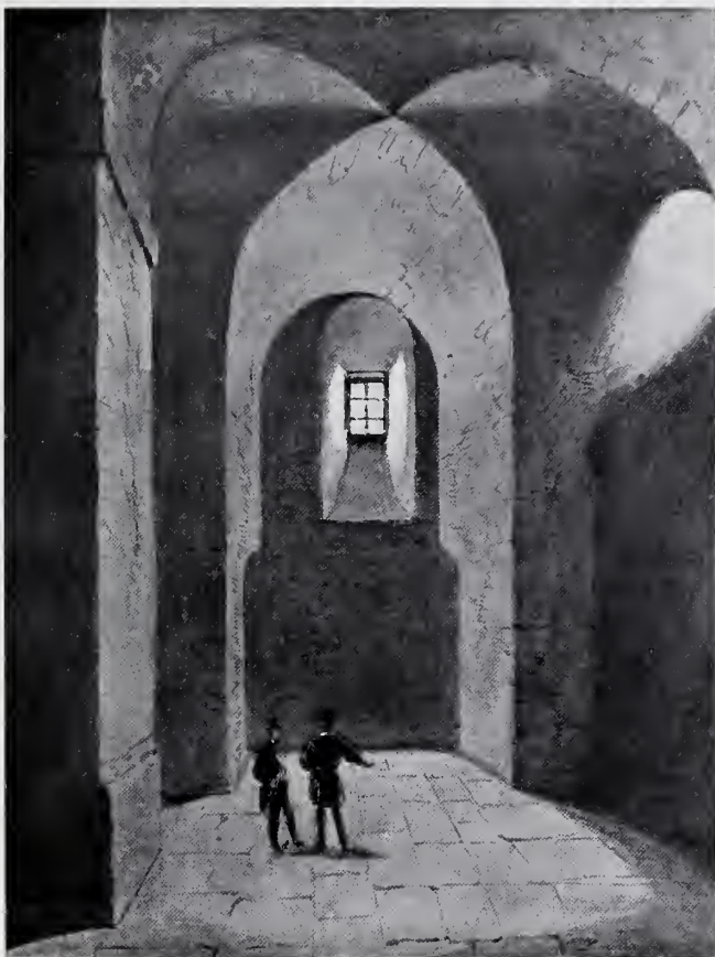
17. VAULTED ROOM IN THE CRYPT OF THE WHITE TOWER, IN WHICH THE RACK STOOD. From a drawing in the Gardner Collection.
