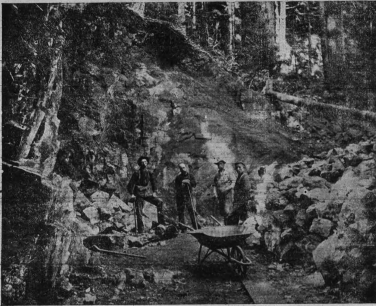
OLYDE'S CUT, COMSTOCK MOUNTAIN—SHOWING METHOD OF QUARRYING OIL ORE ON YREKA PROPERTY. PART OF THE DUMP IS SEEN, ALL TO LEFT IS ORE.
