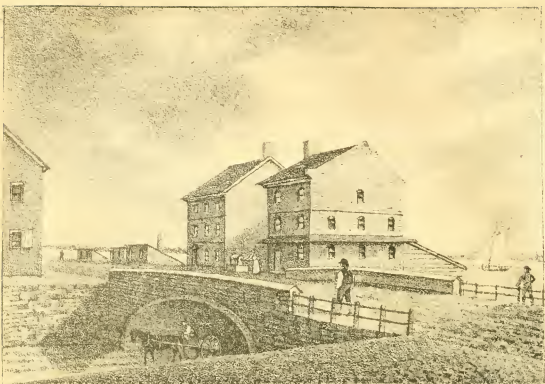
Arch Street Bridge, at Front Street
