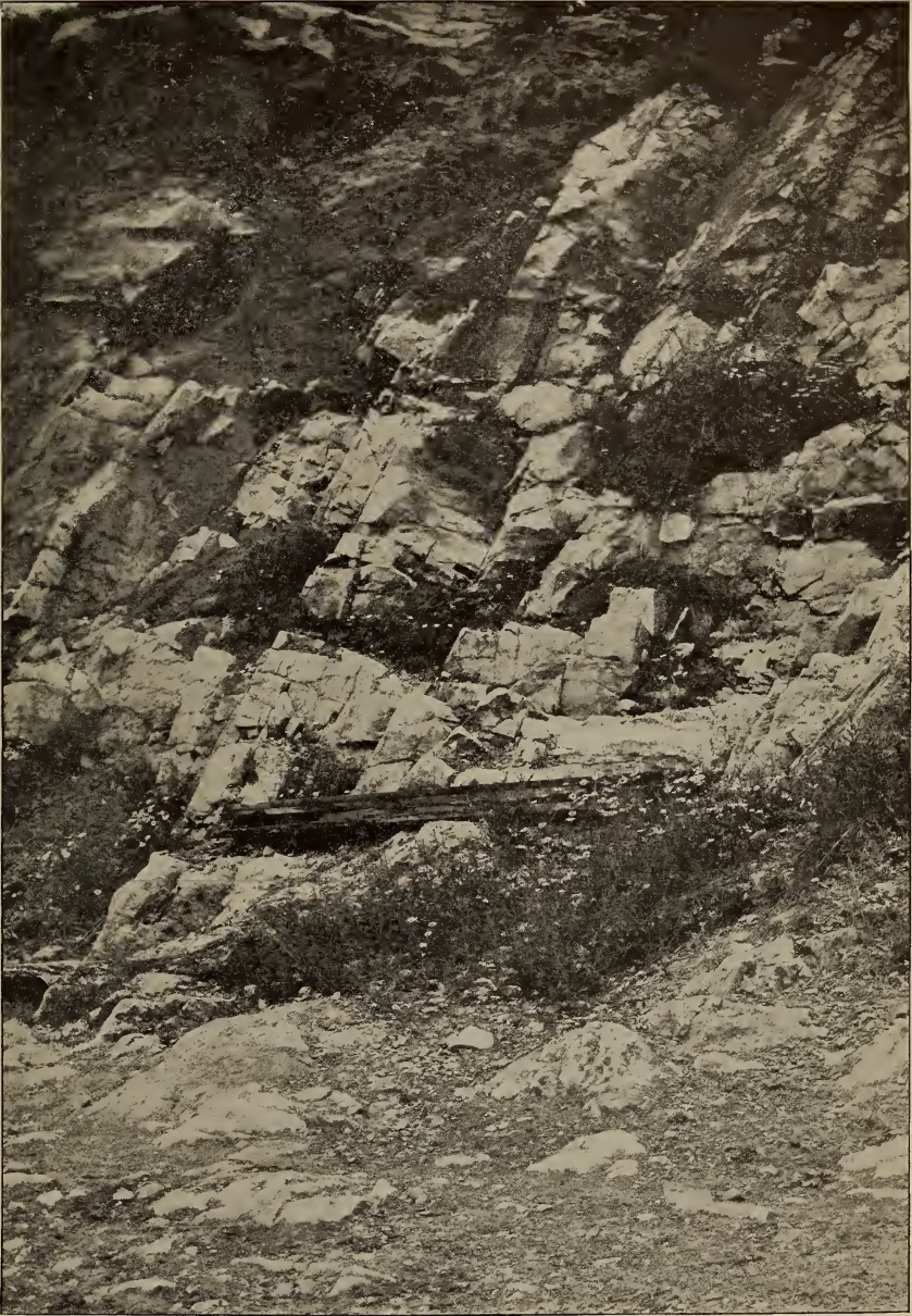
Road metal quarry in Grenville limestone at Theresa near the falls. The limestone bed is a thin one in the general schist series and the quarry face is down the dip, here 75^{\circ} . At the upper part of the cliff is Potsdam sandstone with irregular contact with the limestone, and showing one of the depressed pockets characteristic of these contacts, filled with weakly cemented calcareous sandstone. H. P. Cushing, photo, 1907
