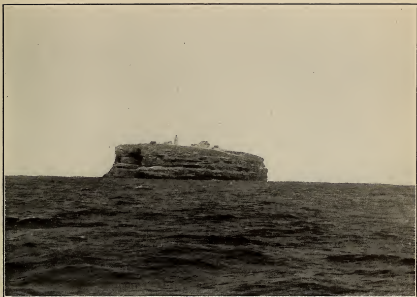
Great Bird rock, from the south; showing light house and accessory buildings
