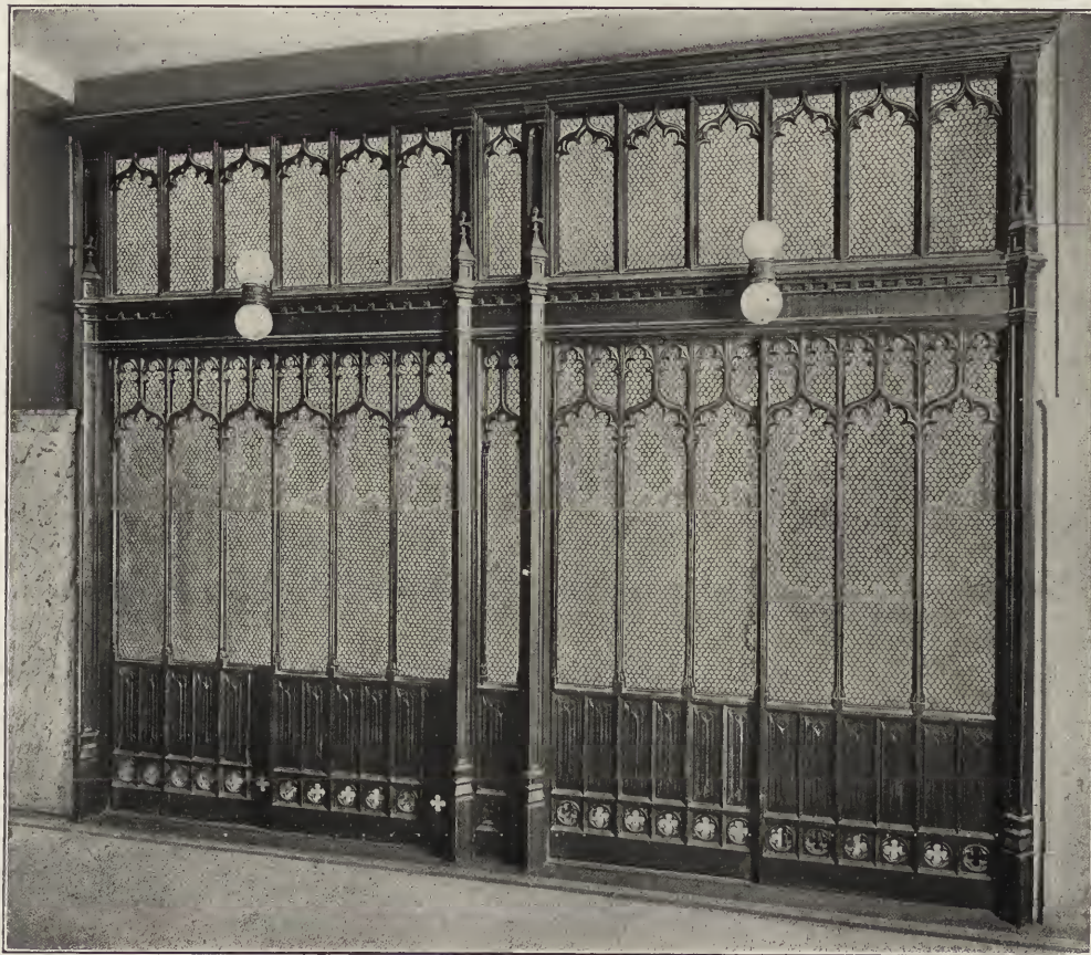
FIG. 4. TYPICAL ELEVATOR ENCLOSURE, 2D TO 23D STORIES, TRINITY BUILDING, 111 Broadway, New York.
