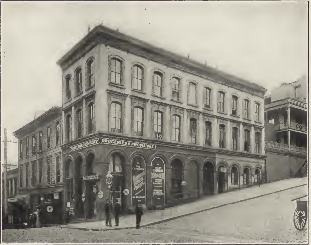
AN INTERESTING BASEMENT ARCADE.
