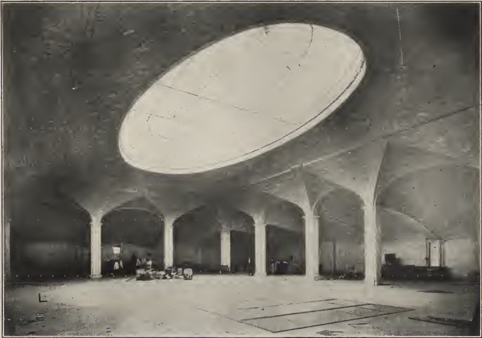
THE HUGE GUASTAVINO VAULT ON THE TOP FLOOR OF TIFFANY & CO.'S BUILDING. Fifth Avenue and 37th Street, New York.
