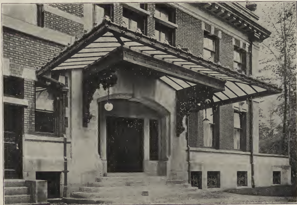
RESIDENCE OF LOFTUS CUDDY, ESQ.—DETAIL OF CARRIAGE ENTRANCE. Cleveland, O. J. Milton Dyer, Architect.
