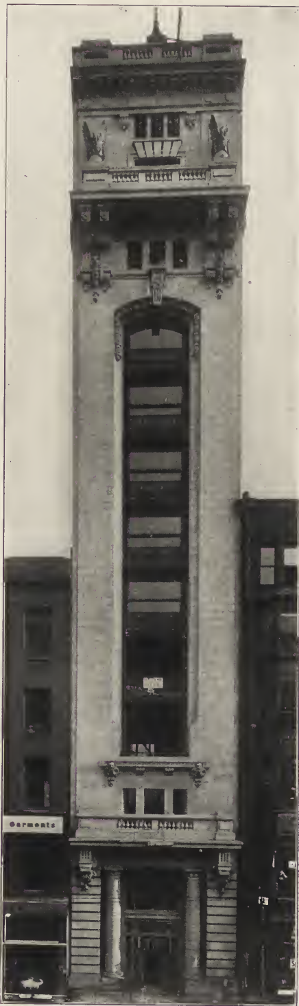
GUARDIAN SAVINGS AND TRUST CO. Cleveland, O. J. Milton Dyer, Architect.
