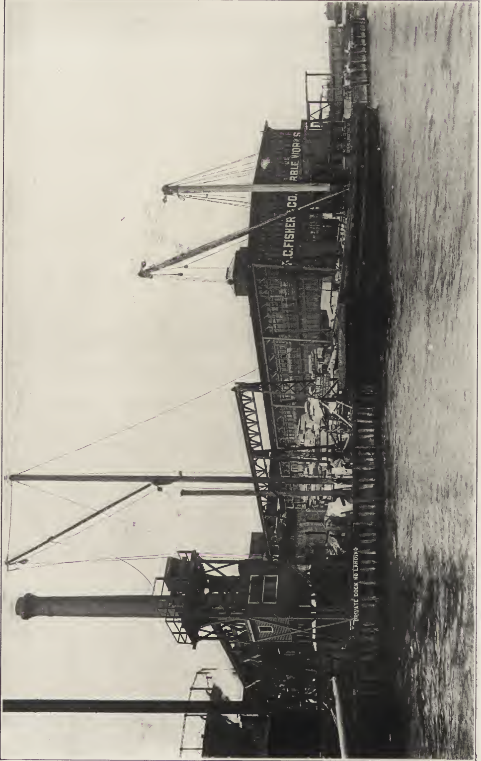
THE ROBERT C. FISHER CO., MARBLE WORKS, NEW YORK CITY. General View from the East River.
