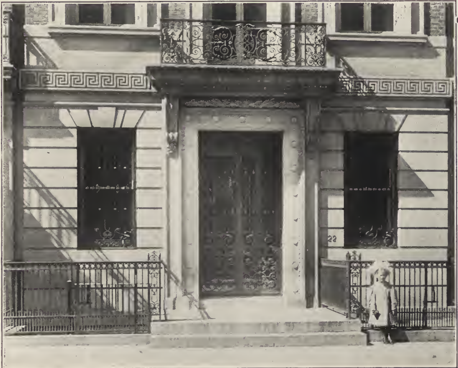
THE CLARK ESTATE HOUSES—DETAILS.
