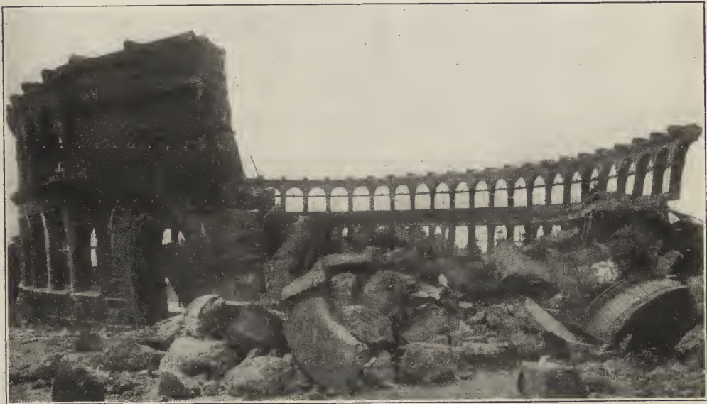
"THE PANORAMA," A CONCRETE STRUCTURE WRECKED BY THE EARTHQUAKE. Golden Gate Park, San Francisco, Cal.
