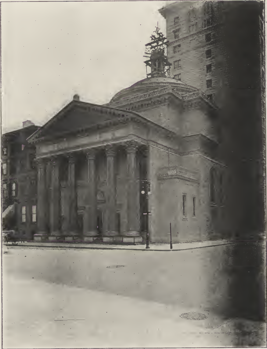
THE MADISON SQUARE PRESBYTERIAN CHURCH. Madison Avenue and 24th Street, New York.
