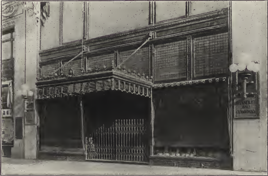
FIG. 8. A RICHER BUT LESS SUCCESSFUL MARQUISE: THE CHANDLER STORE BUILDING. Boston, Mass. Peabody & Stearns, Architects.
