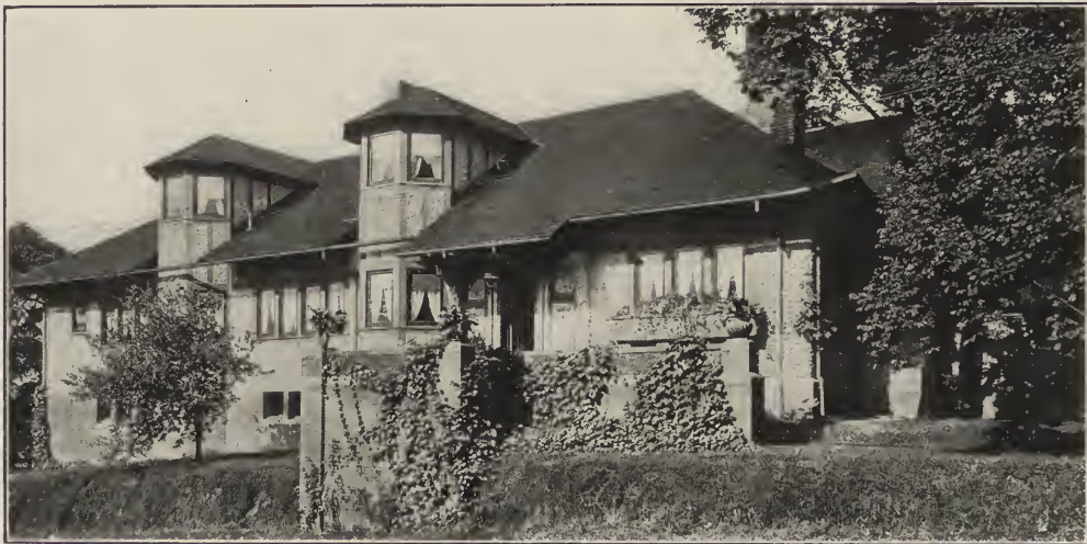
FIG. 1. MRS. WATERMAN'S HOUSE AT PARKERSBURG, WEST VIRGINIA.
