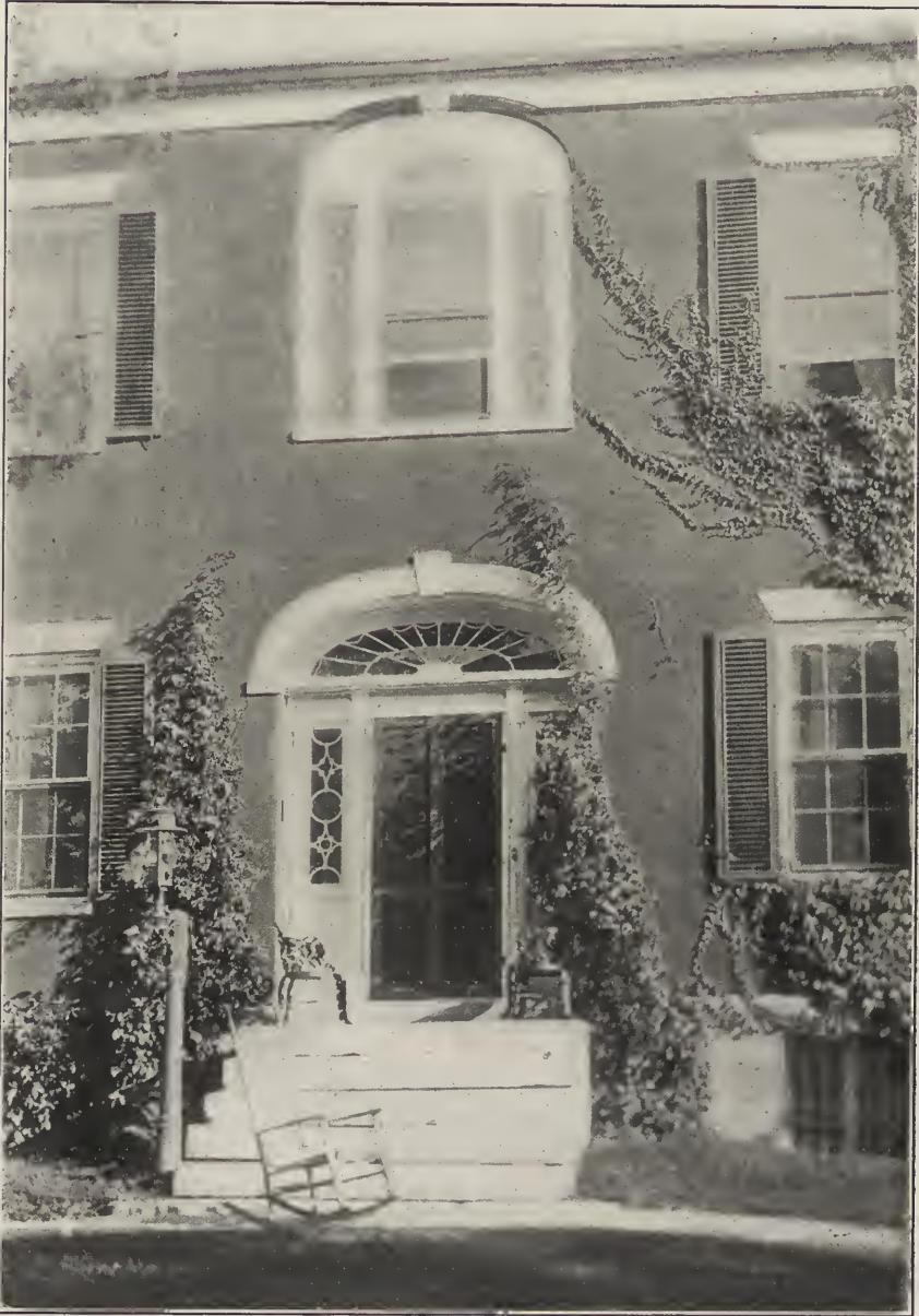
DETAIL OF STOOP—HOUSE OF COMMODORE ELISHA CAMP. Sackett's Harbor, N. Y.
