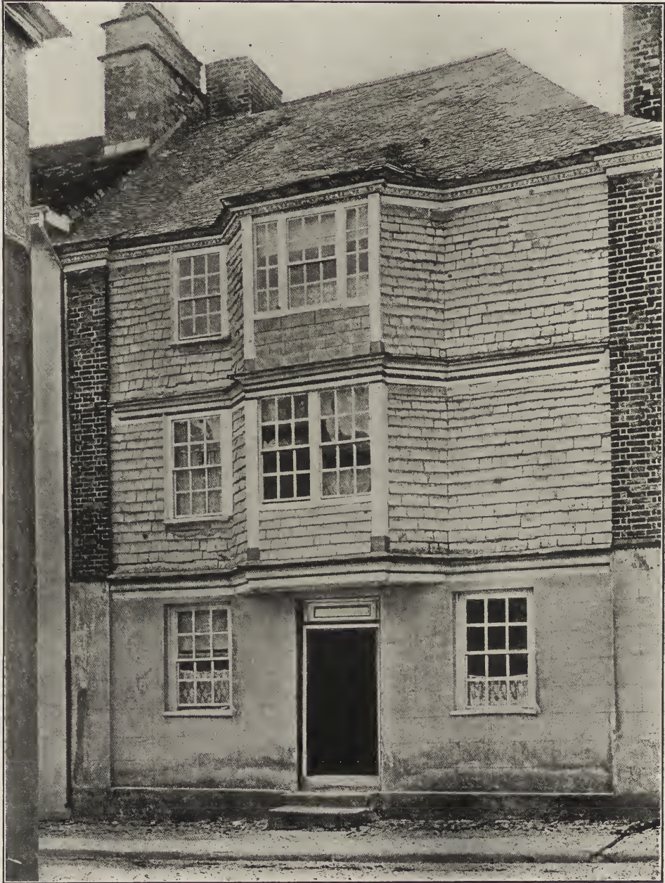
FIG. 10. HOUSE AT ASHBURTON. Slating replaces weather-boarding.
