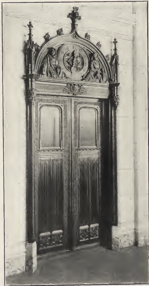
Fig. 3. Bronze and Wire Glass Elevator Doors on the First Story of the Trinity Building, 111 Broadway, New York.
