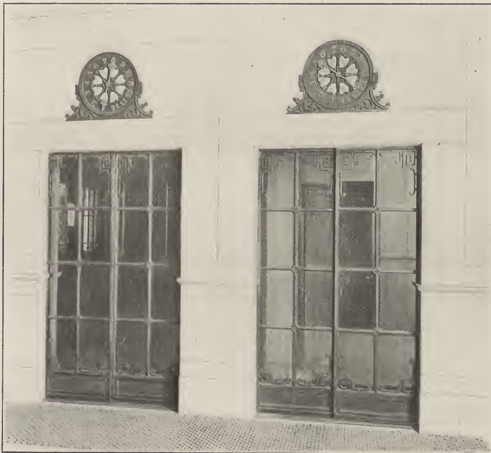
FIG. 5. A FRANK BUT DECORATIVE TREATMENT OF AN IRON AND WIRE GLASS ELEVATOR ENCLOSURE. THE RECTOR BUILDING.
