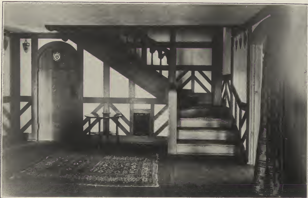
FIG. 6. MR. GRAFTON ST. L. ABBOTT'S HOUSE—THE STAIR HALL. Concord, Mass. (Photo by M. H. Northend.) Philip B. Howard, Architect.
