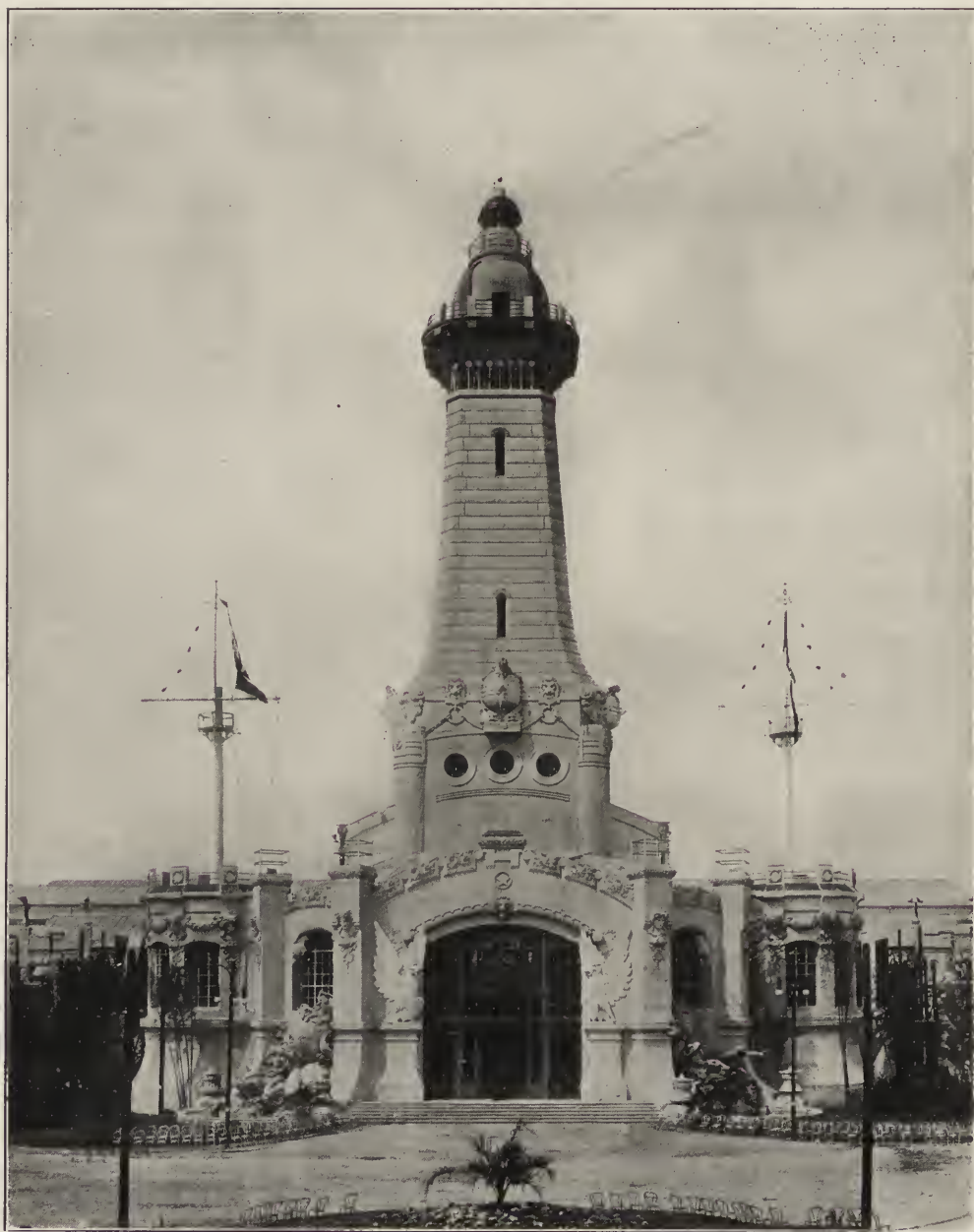
MARINE TRANSPORT, MAIN FRONT AND LIGHTHOUSE.
