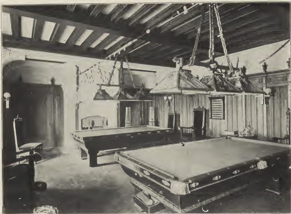
CONVERSE MANOR, THE ESTATE OF MR. E. C. CONVERSE—THE BILLIARD ROOM. Greenwich, Conn. Donn Barber, Architect. (Photo by Alman & Co.)
