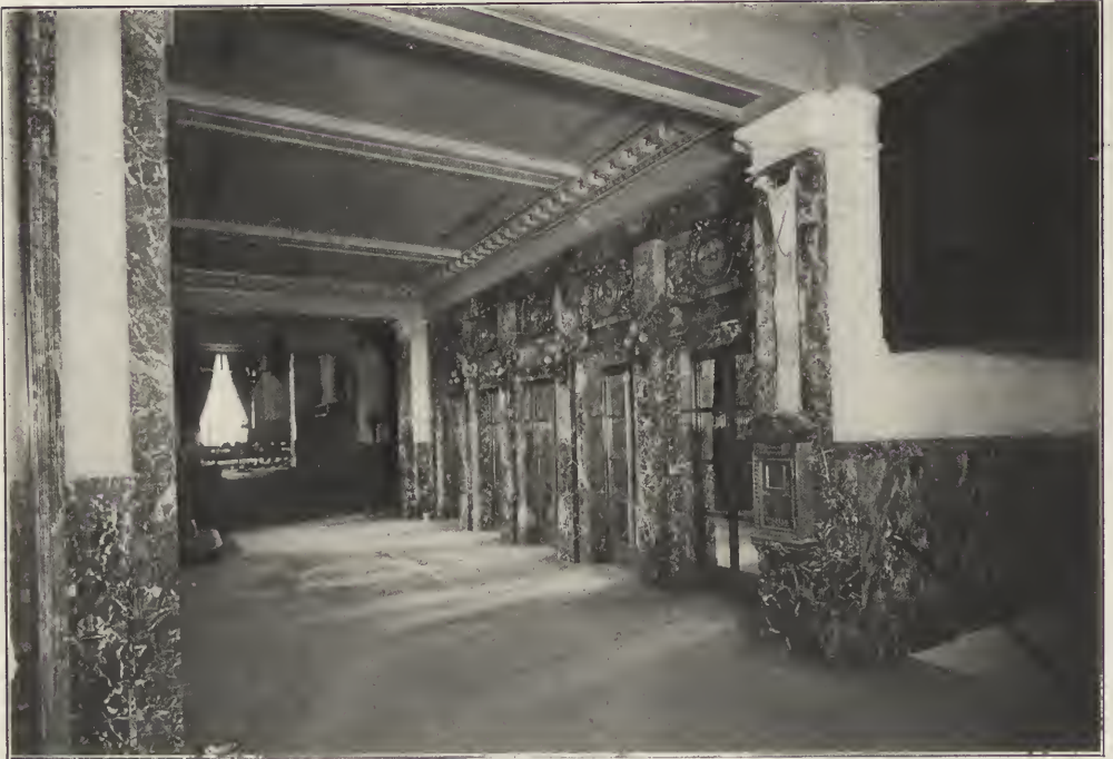
FIG. 5. THE ELEVATOR ENCLOSURES ARE TREATED IN MARBLE AND THE DOORS ARE COVERED WITH MIRRORS—HOTEL BELMONT. Park Avenue, 41st and 42d Streets, New York. Warren & Wetmore, Architects.
