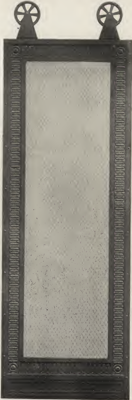
Fig. 2. Iron and Wire Glass Elevator Door, Kean, Van Cortlandt Building, New York, N. Y.
