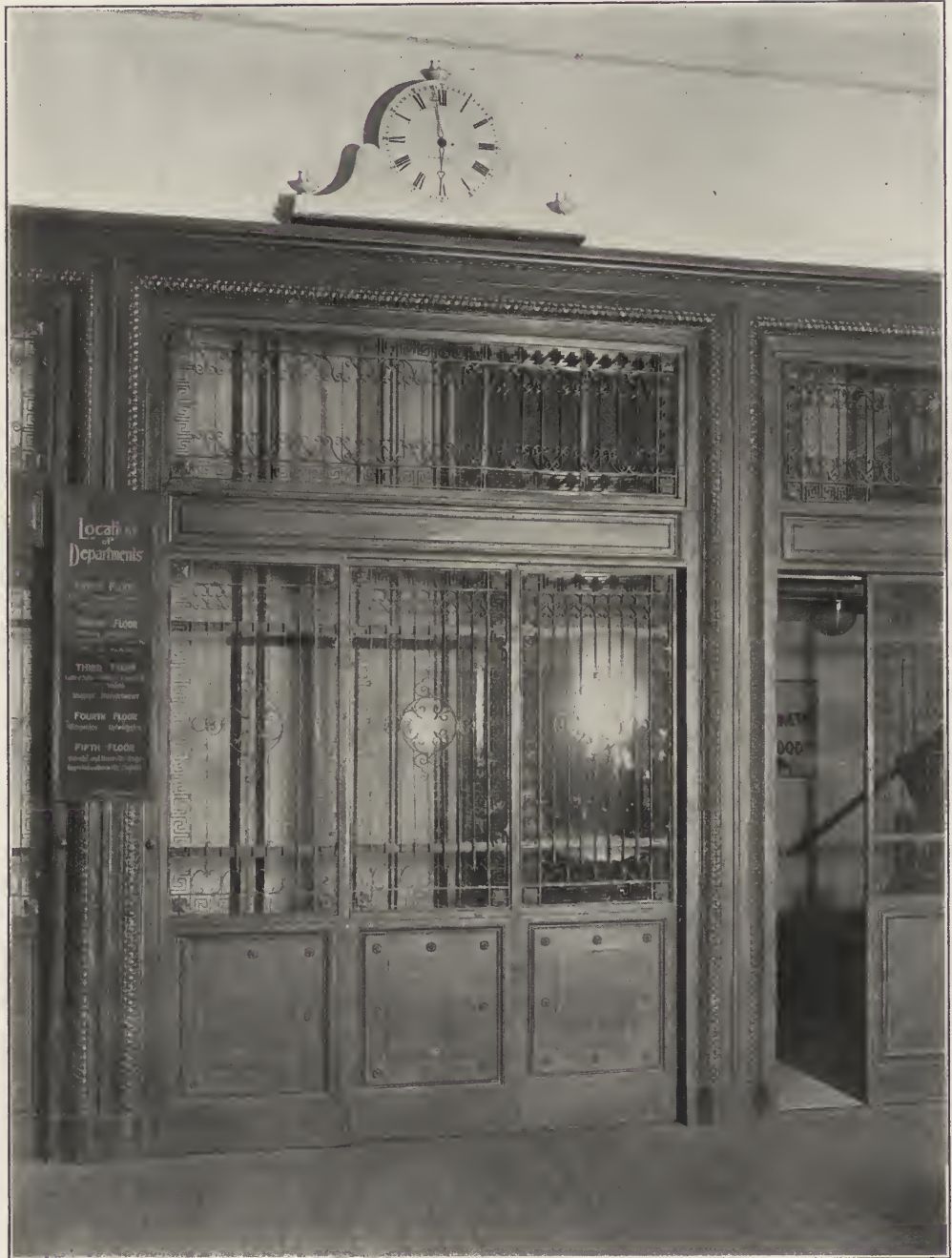
FIG. 6. A MORE ELABORATE METAL DECORATION WITH LESS GLASS SURFACE THAN FIG. 5. CHANDLER STORE BUILDING. Boston, Mass. Peabody & Stearns, Architects.
