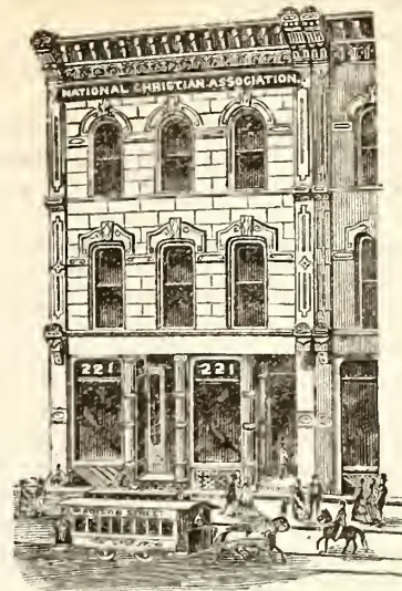
N. C. A. BUILDING AND OFFICE OF THE CHRISTIAN CYNOSURE, 221 WEST MADISON STREET, CHICAGO
