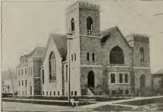
ST. STEPHEN'S CHURCH, WINNIPEG.
