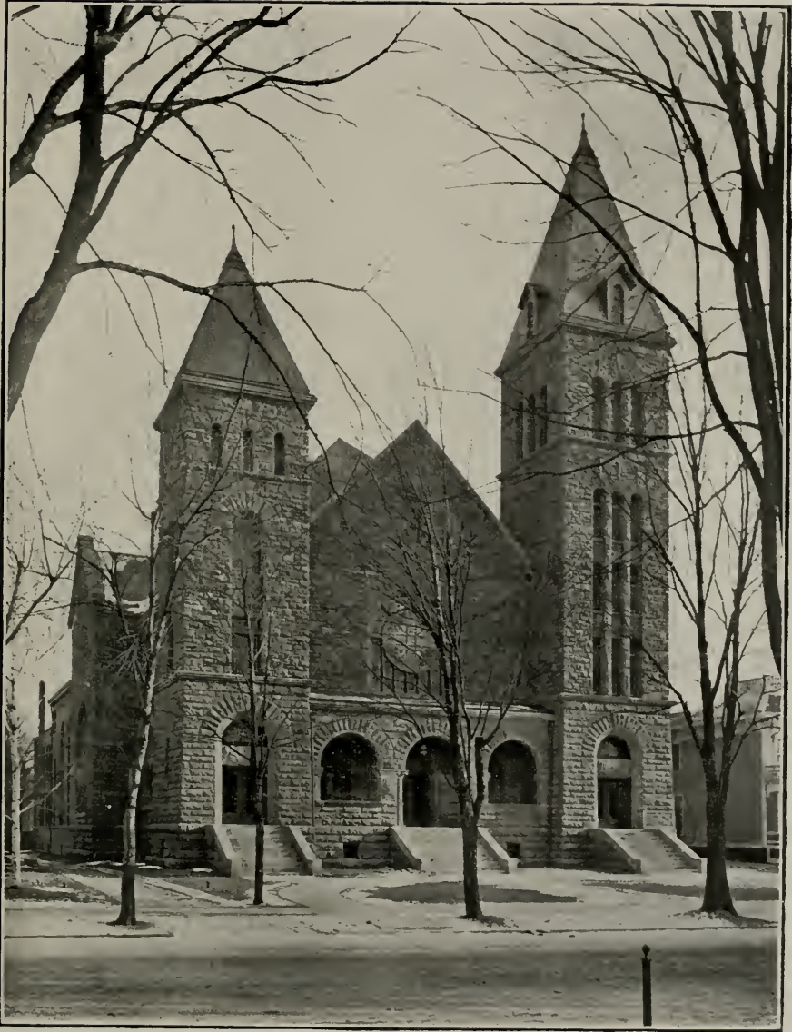
DELAWARE AVENUE BAPTIST CHURCH, BUFFALO.
