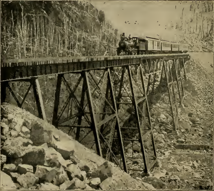
Viaduct on Moosehead Lake Division, B. & A. R. R., built by the Pennsylvania Steel Company.
