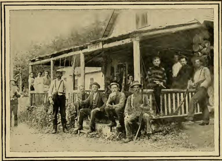
A Typical Camp Assemblage.
