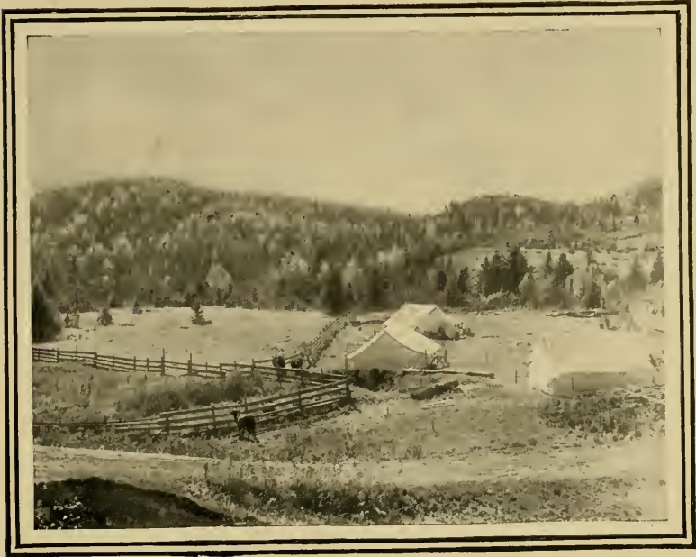
Railroad Surveyors' Quarters.
