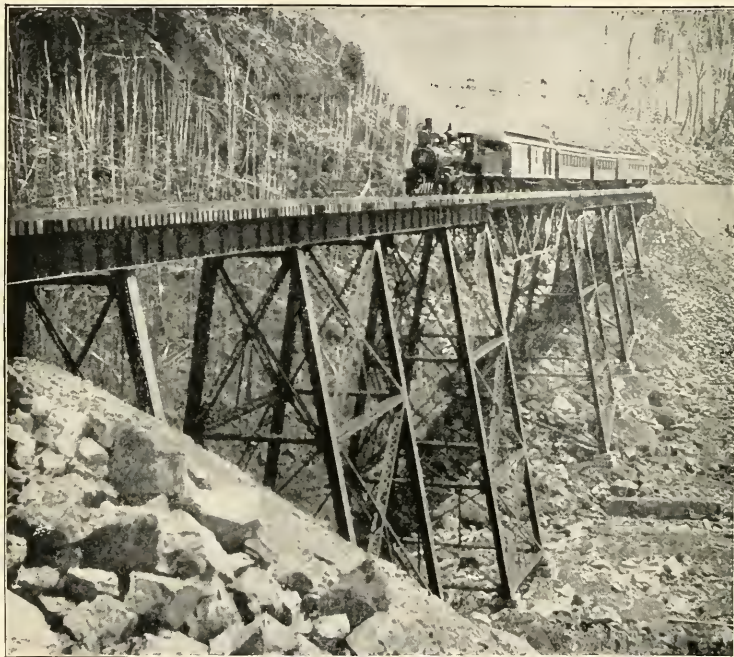
Viaduct on Moosehead Lake Division, B. & A. R. R., built by the Pennsylvania Steel Company.
