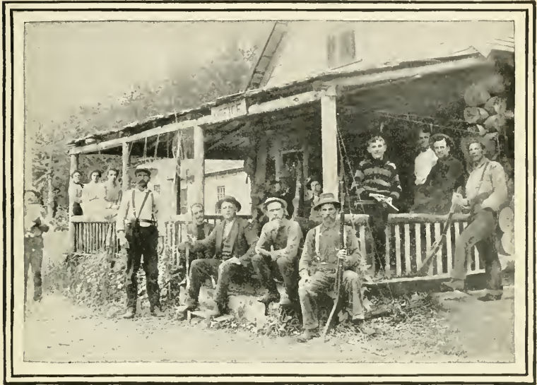
A Typical Camp Assemblage.
