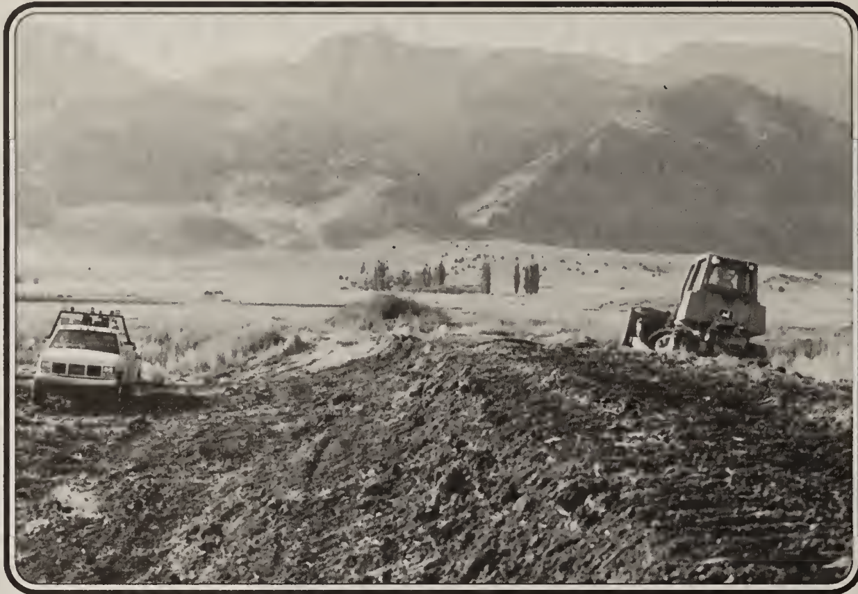
Dike construction in the Warner Wetlands.
