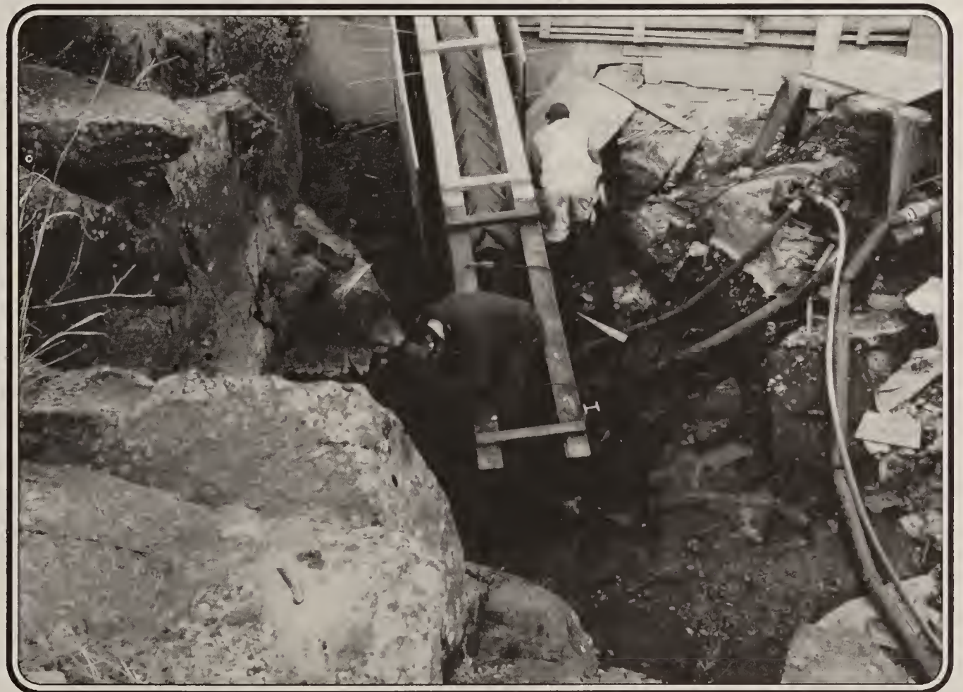
Construction of the Twentymile Creek Fishway.
