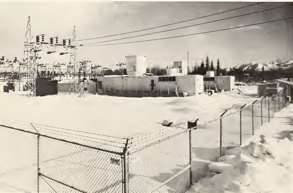
Packaged diesel units, right, or gas turbines, below, are used to generate power in remote Alaskan villages. Isolation and extreme weather conditions make long-distance transmission lines impractical.
