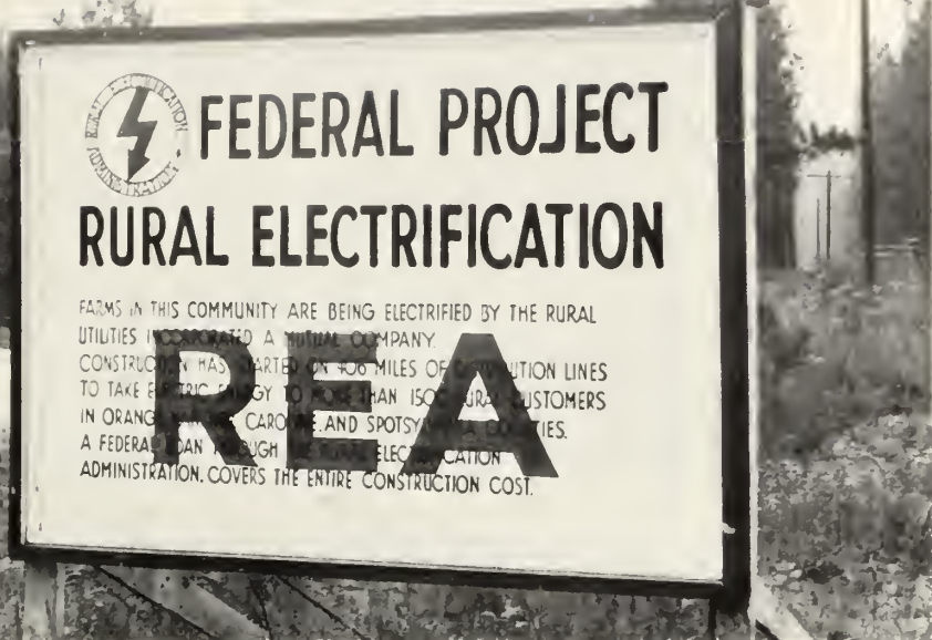
Early REA sign let local people know electricity was on the way.
