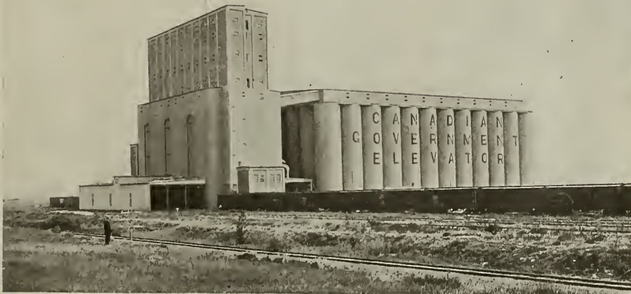
THE 3,500,000-BUSHEL CANADIAN GOVERNMENT ELEVATOR AT SASKATOON, SASK. The Government Elevator at Moose Jaw is a Duplicate of This House
