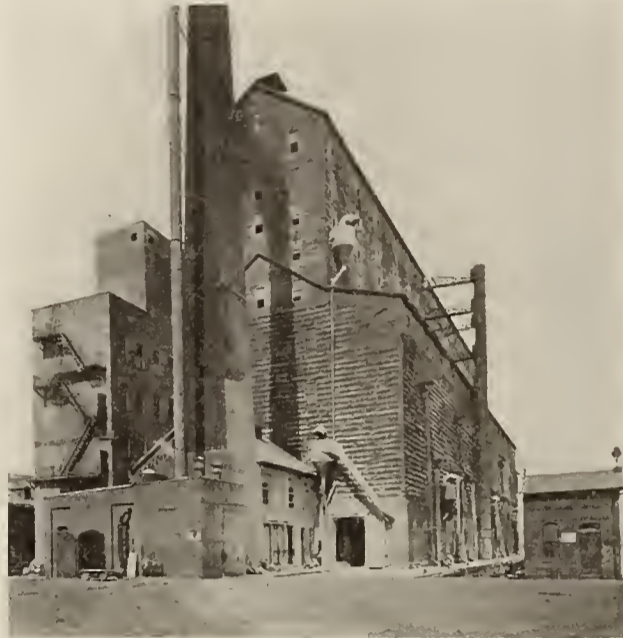
ELEVATOR B Showing dust collectors from cleaners and sweep up systems
