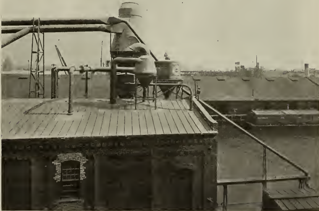
ROOF OF THE DUST HOUSE
