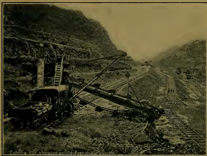
CULEBRA CUT. PART OF THE OLD FRENCH EXCAVATION.
