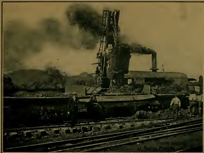
A STEAM SHOVEL AT WORK ON THE CANAL.
