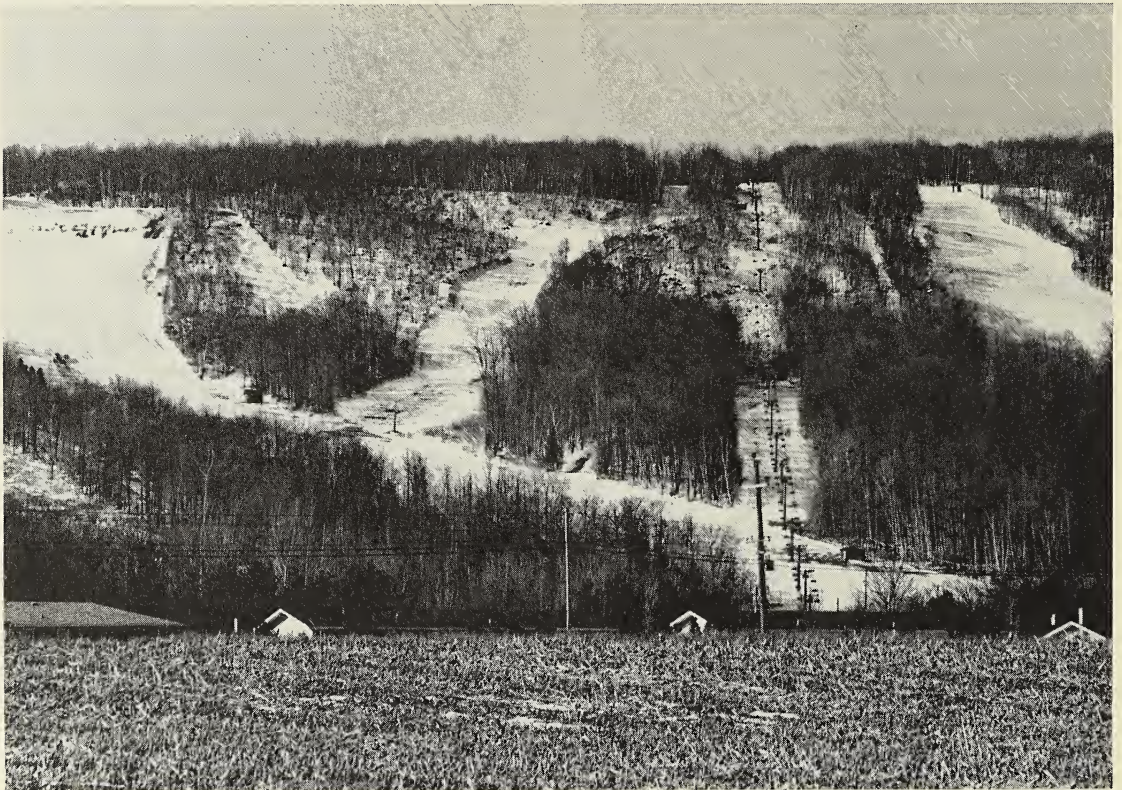
Fig. 6. Rib Mountain Ski Area, from the north.
