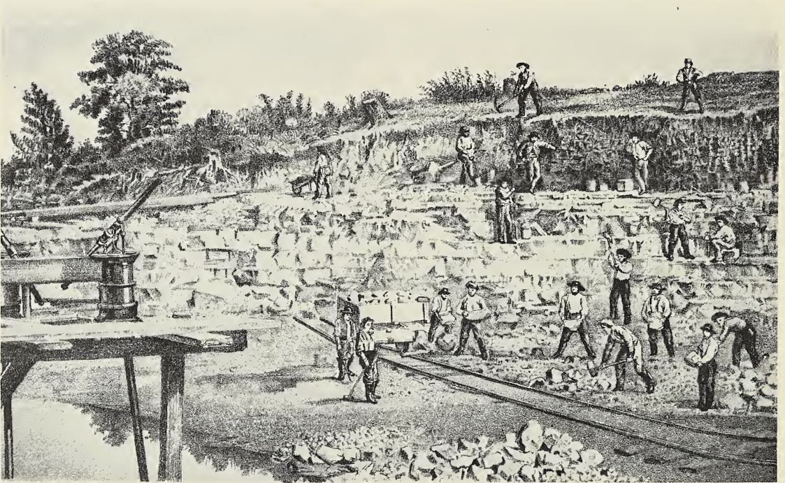
Fig. 2. Lithograph demonstrating typical nineteenth century quarrying methods. Quarry depicted was in Devonian rocks at Mill No. 1 of the Milwaukee Cement Company shortly after the company began operations, ca. 1876. The area shown in the lithograph is on the east bank of the Milwaukee River, near the old swimming beach in Estabrook Park, Milwaukee. From Chamberlin (1877); drawn from a photo taken by J. C. Miller.
