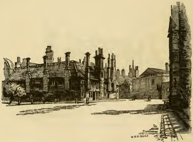
Washhouse Court, Exterior.
