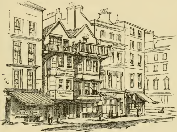
Drayton's House, Fleet Street.
