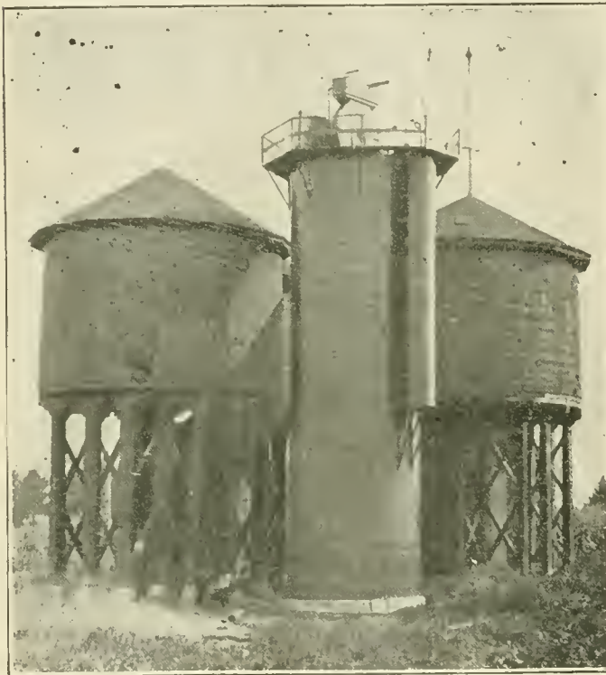
Water Service on the Chicago, Burlington & Quincy.
