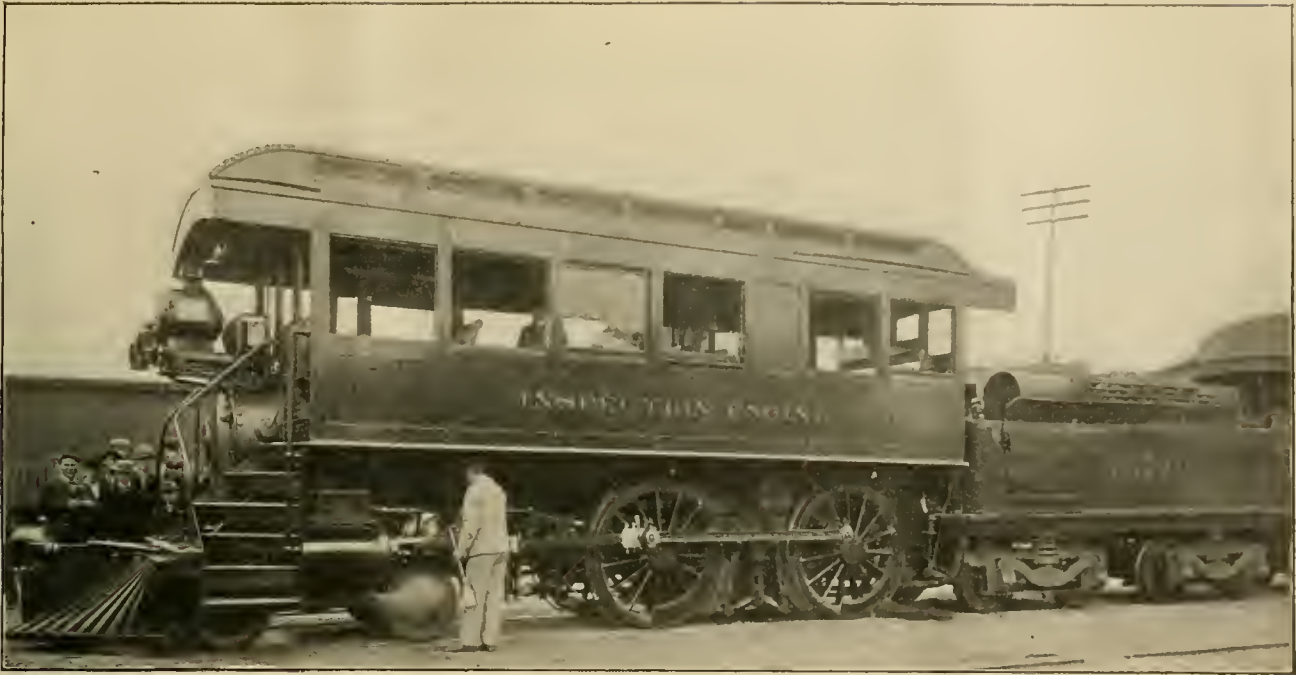
Inspection Locomotive—Chicago, Burlington & Quincy Railroad.
