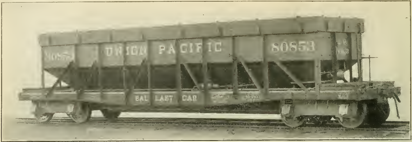
Fifty-Ton Ballast Car—Union Pacific Railway.
